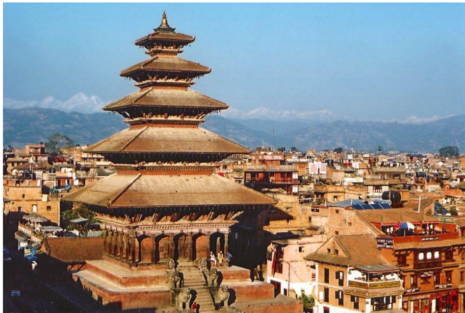
Figure 3.1: View of Nyatapola Temple in Bhaktapur, Nepal (Chandra Niraula 2016).
