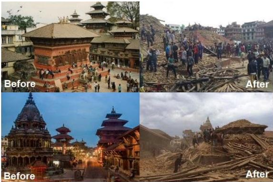
Figure 3.10: Examples of the cultural heritage sites in Kathmandu and Patan Durbar Squares destroyed by Gorkha earthquake, 2015 (Nepal Current News 2015)
