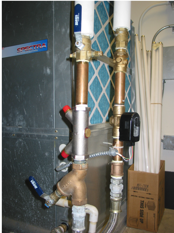
Figure 5.11. New heat pump connection piping configuration.
