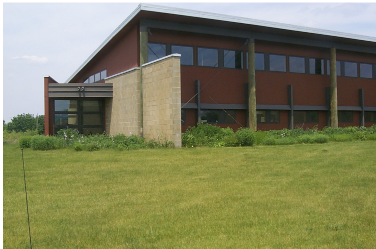
Figure 3.5. Southwest corner of the IAMU's north wing. Notice the many exterior shading devices. (John Burnet, IAUM)
