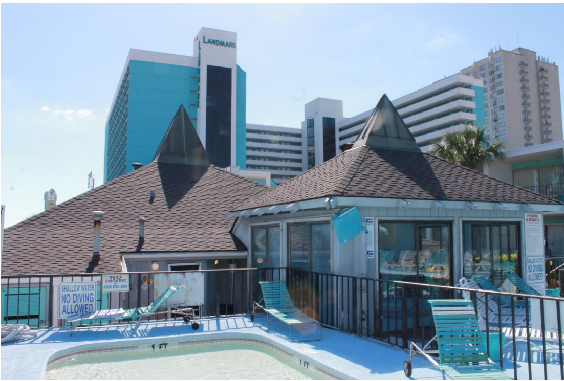
Figure 2.17 Sliding doors on additional hut. (Photo by the author.)
