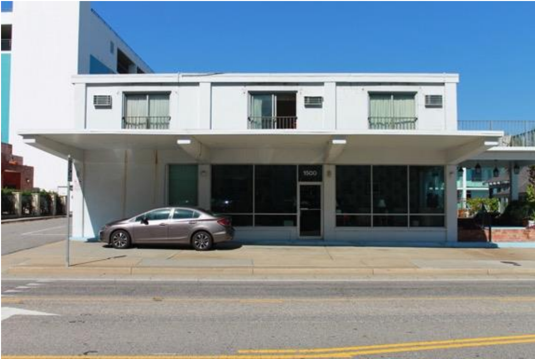
Figure 2.2 South end of east elevation, front office. (Photo by the author.)
