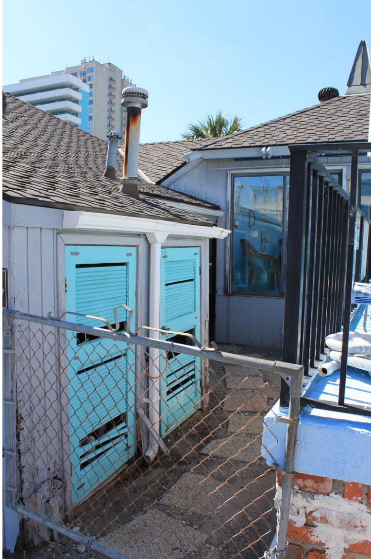
Figure 2.15 Shed addition on hut for pool equipment. (Photo by the author.)
