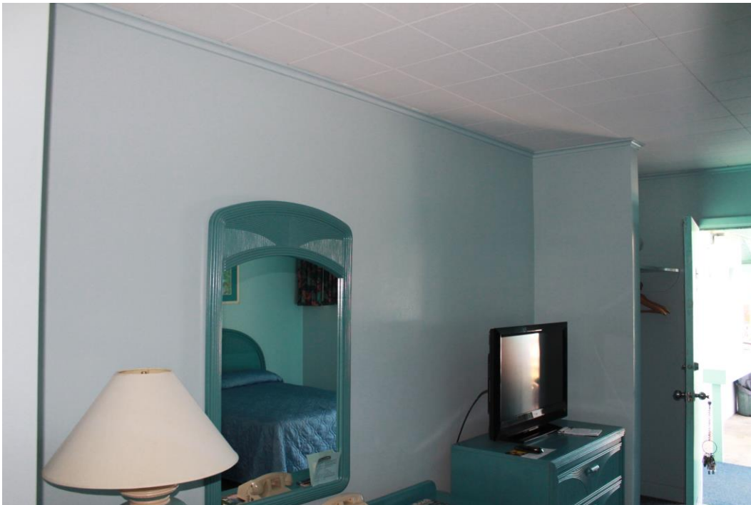
Figure B.3 Current sheetrock wall. (Photo by the author.)
