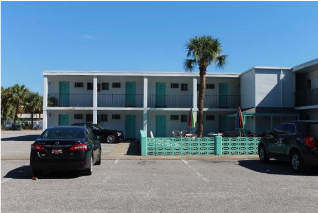
Figure 2.10 South elevation of 1967-1969 addition. (Photo by the author.)
