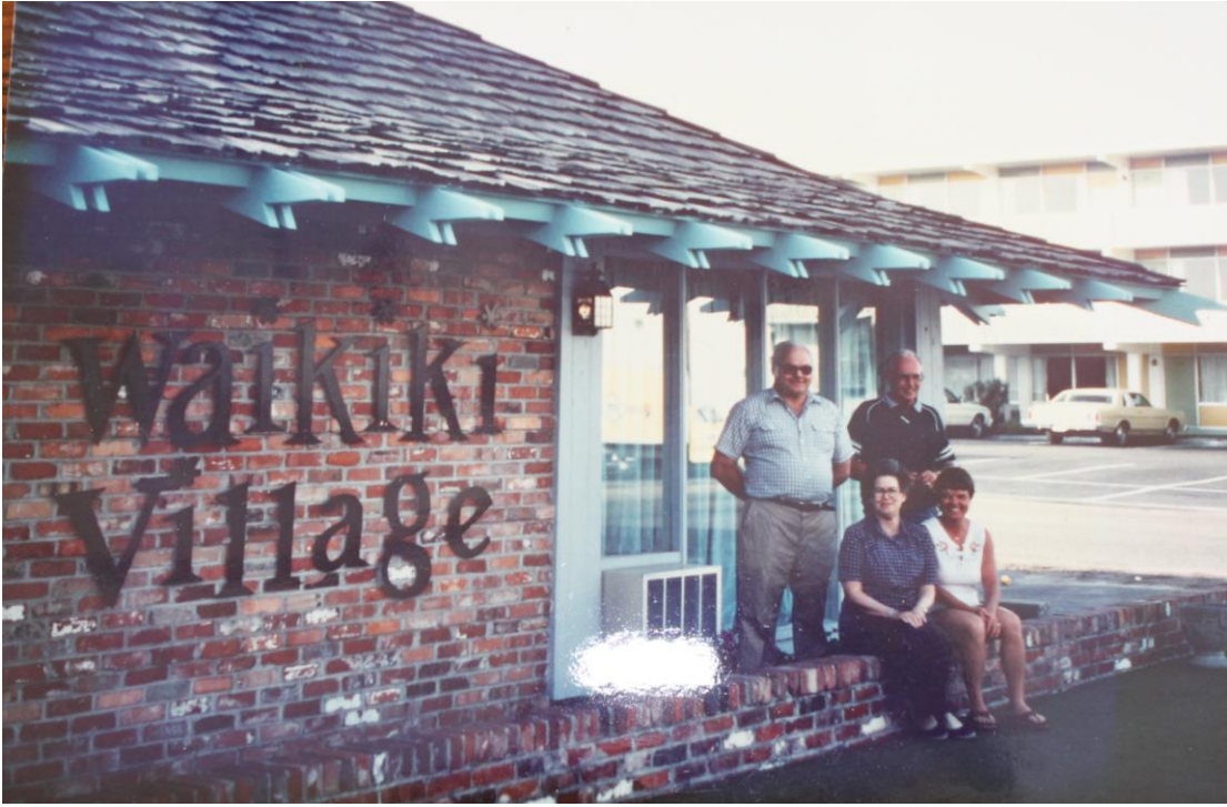
Figure 2.32 Original exposed rafter tails. (Photo courtesy of Nancy Watts Hall.)
