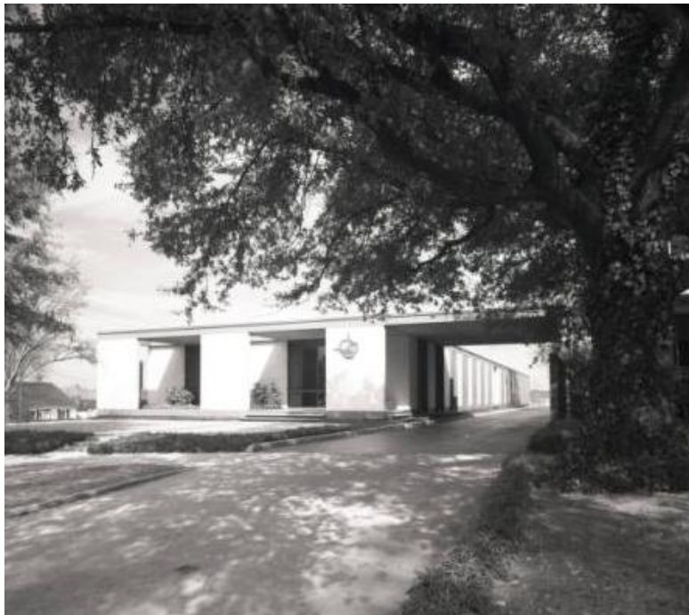
Figure 2.5. 1800 Gervais Street Office. From an unknown source, WFA.
