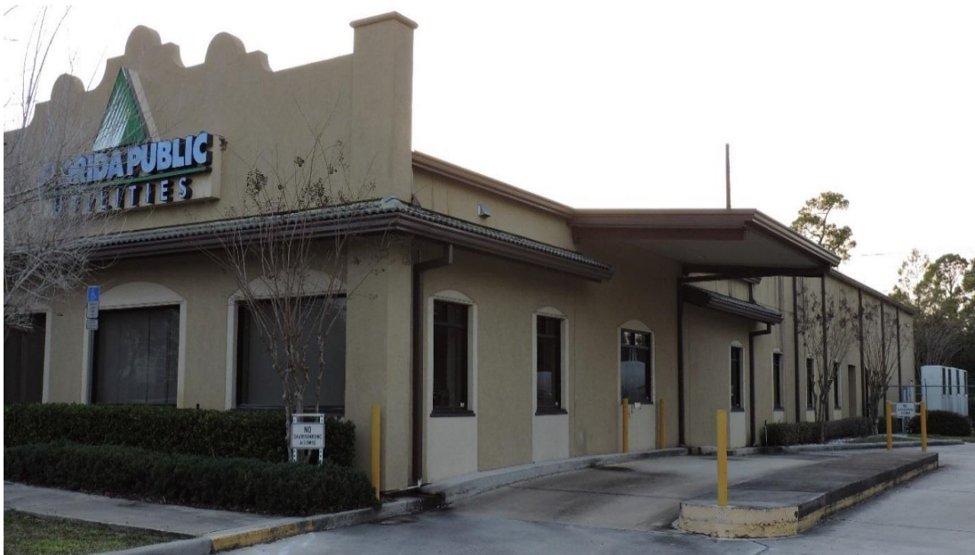
Figure 10. Office building of Florida Public Utilities, Debary, FL
