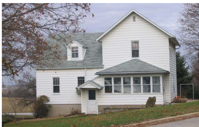
Figure 6. The first school building (AS2).
