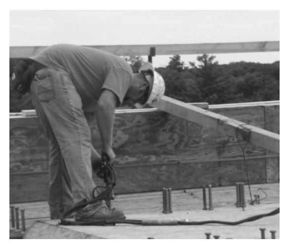
Figure 38. Posture maintained during traditional stud welding
