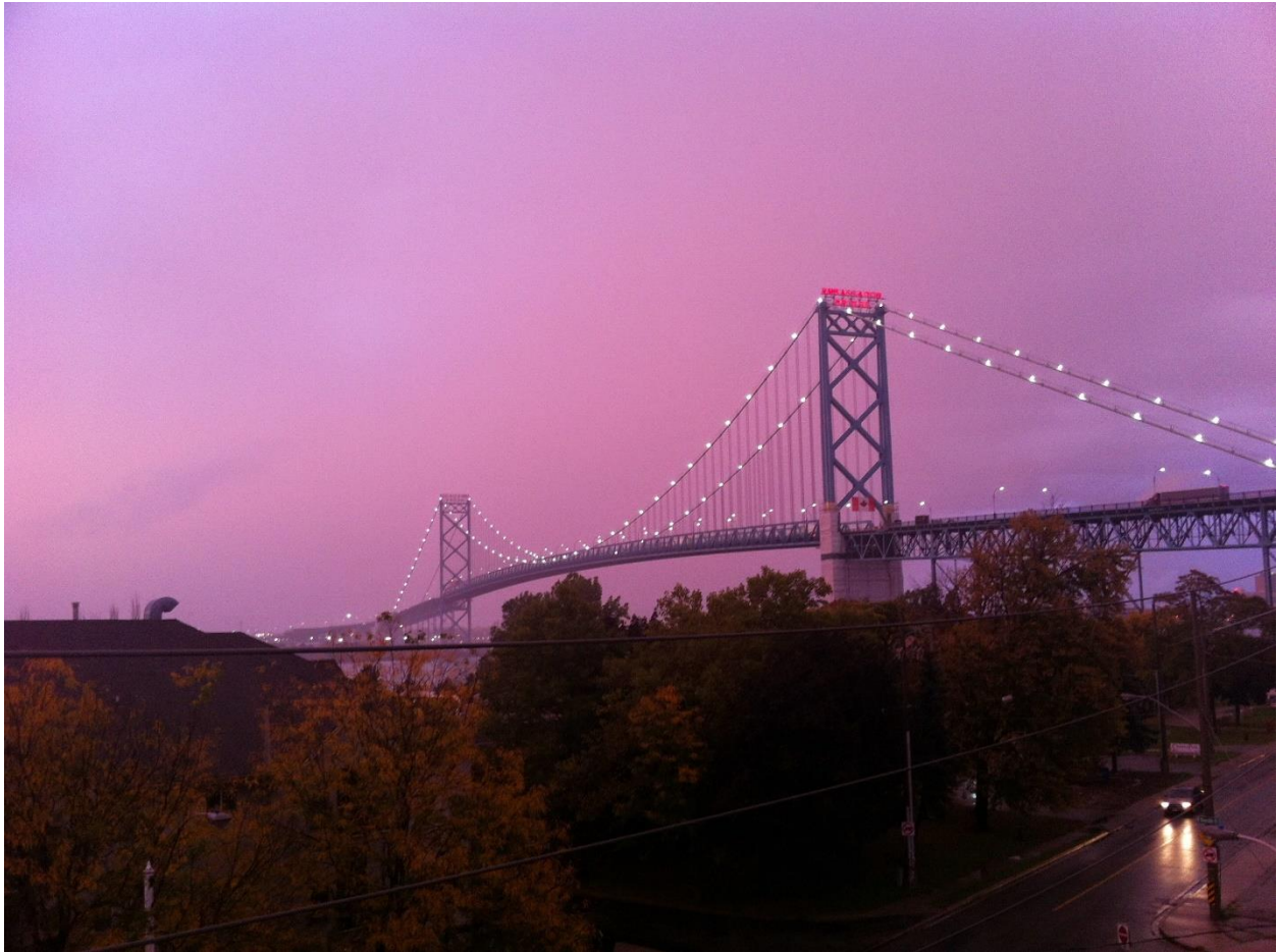
Figure 1 - Ambassador Bridge, Windsor, ON, Canada
