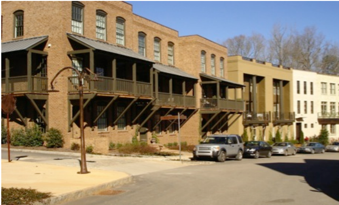
Figure 18 The first phase of construction at Serenbe.
