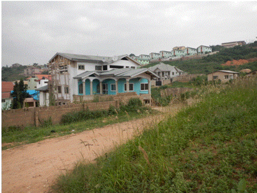
Figure 6. Housing in Ashongman Estates
