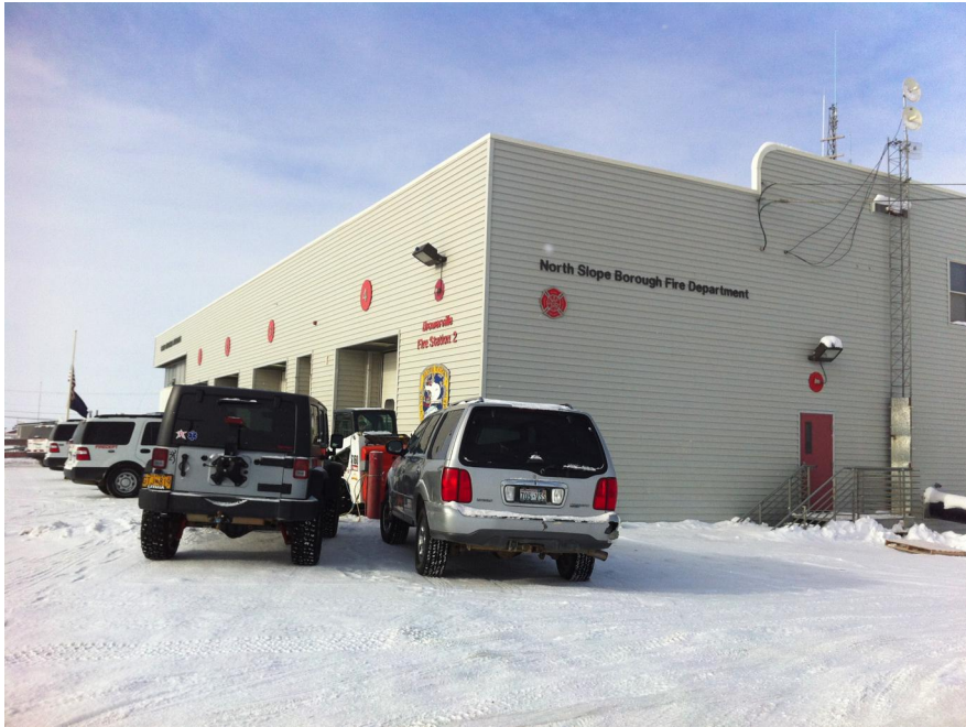
Figure 3. New municipal building and service vehicles in Barrow, NSB. March 2015. (G Parente).
