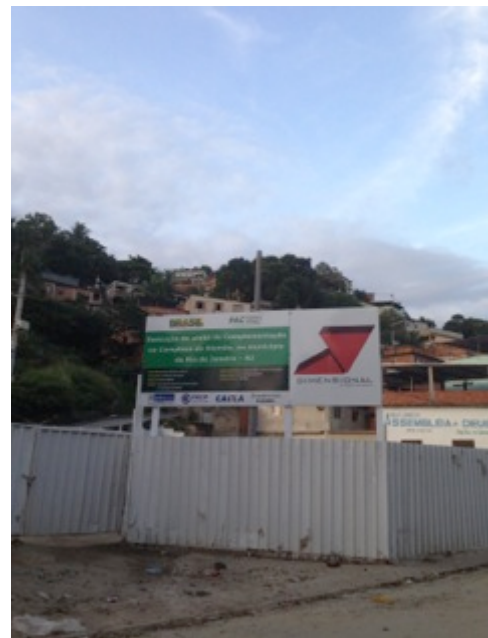
Figure 3.4 PAC construction in Complexo. Photo taken 21 Apr 2014 by author.
