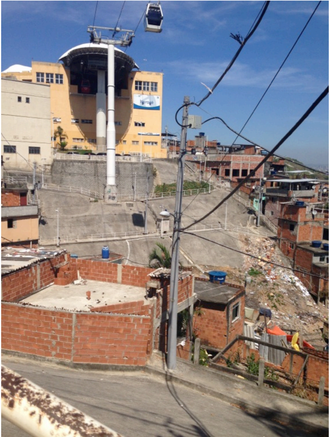
Figure 1.4 Itararé teleferico station. Photo taken 13 Jan 2014 by author.
