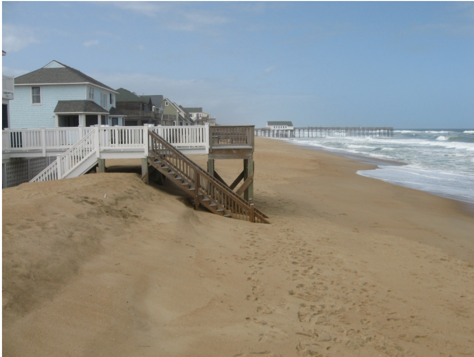
Figure 3.4: Photo taken in March, 2010 of homes being threatened by erosion from recent storms in Kitty Hawk, NC.
