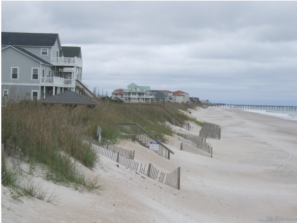
Figure 3.3: Photo of Topsail Island, NC from October, 2009 showing minimal setbacks from the beach (photo courtesy of Dr. Burrell Montz).
