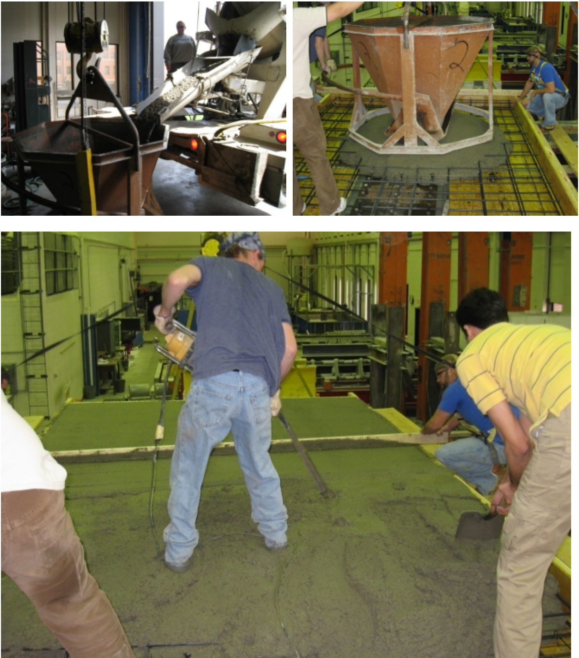
FIGURE 2-9: CONCRETE POURING PROCESS
