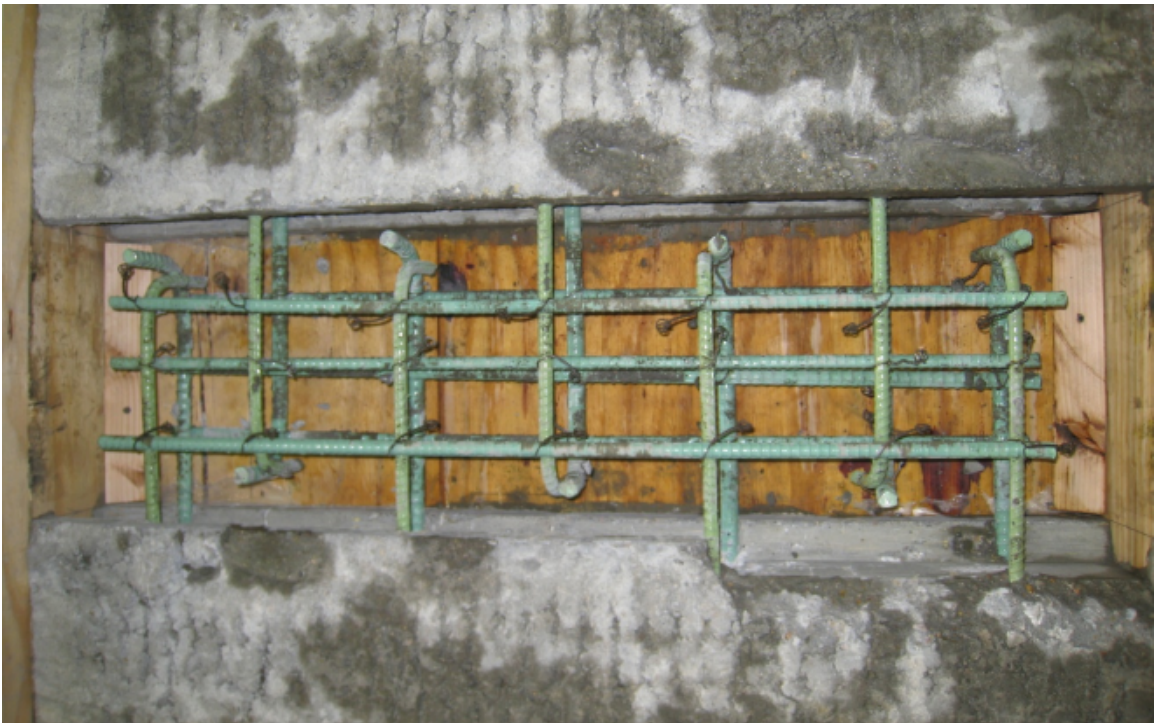
FIGURE 6-8: HOOKED BAR LAB PICTURES
