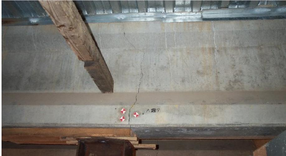
**Figure C30- Cracks near girder supports**
