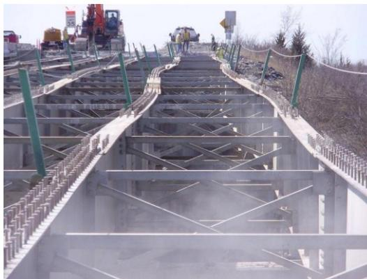
**Figure C62- Improper deck removal**
