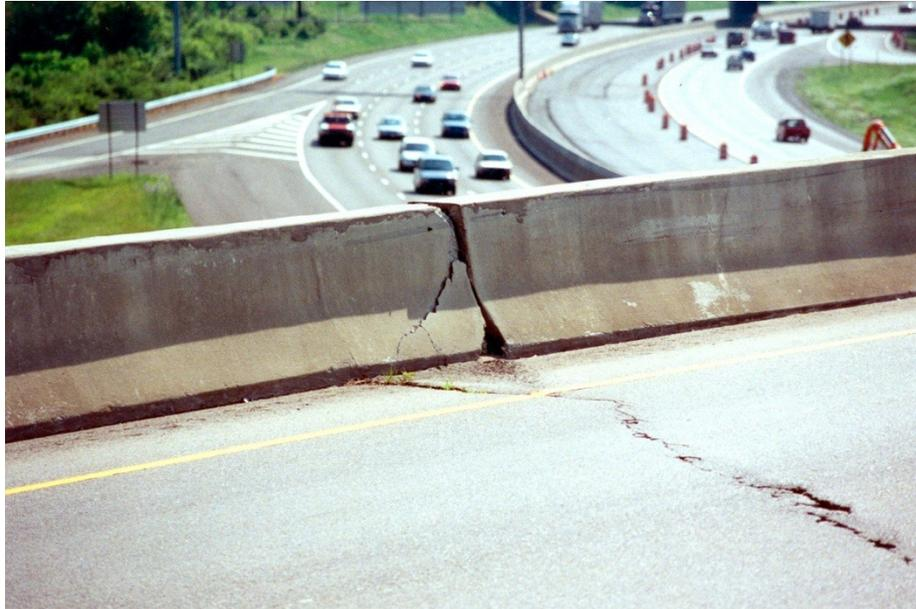
**Figure C20- Barrier distress at west abutment (Tabatabai, Oesterle and Lawson, 2005).**
