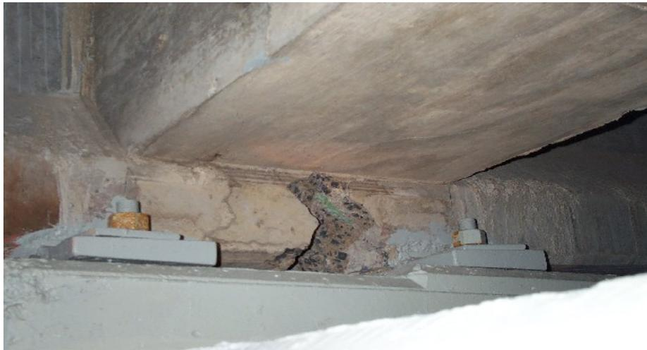
**Figure C31- Crack and spall at diaphragm over pier support**
