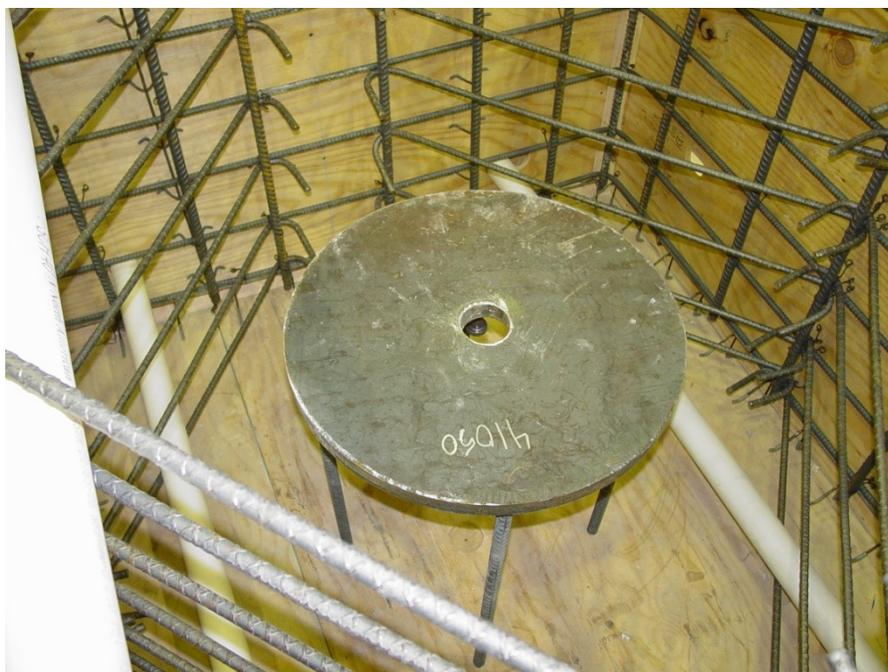
**Figure 4-10- Holding the embedded plate at the middle of the cap**
