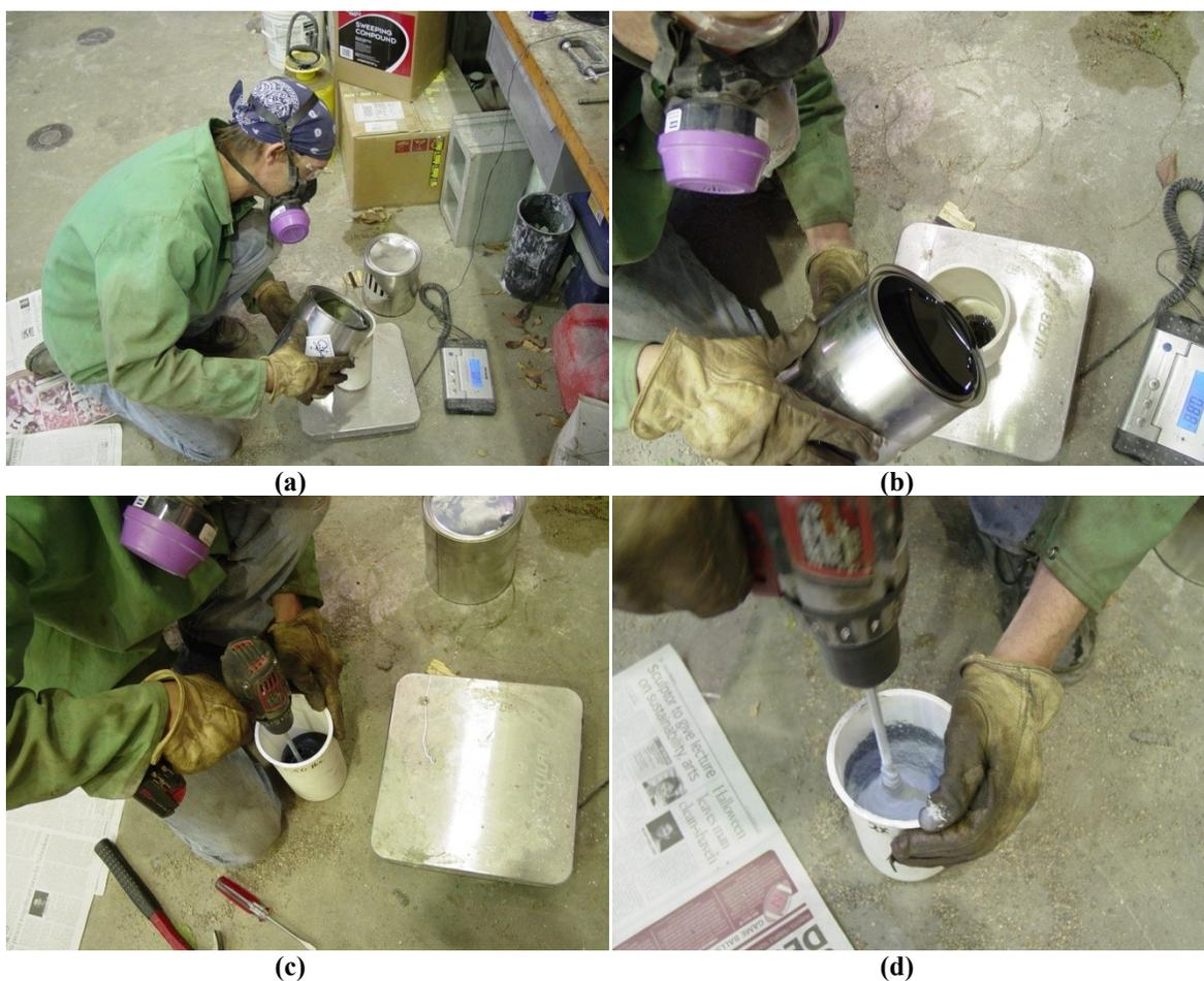
**Figure 4-66- Delpatch mixing procedure**
