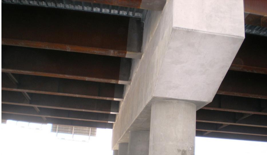
**Figure C49- Integral cap as completed**
