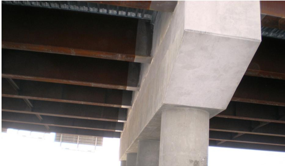
**Figure C49- Integral cap as completed**
