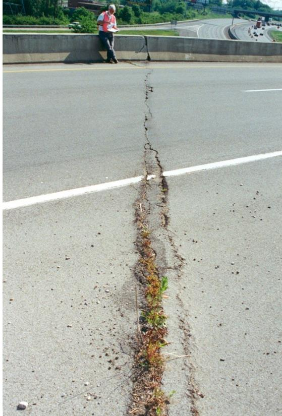
**Figure C19- Asphalt overlay distress (west end) (Tabatabai, Oesterle and Lawson, 2005).**
