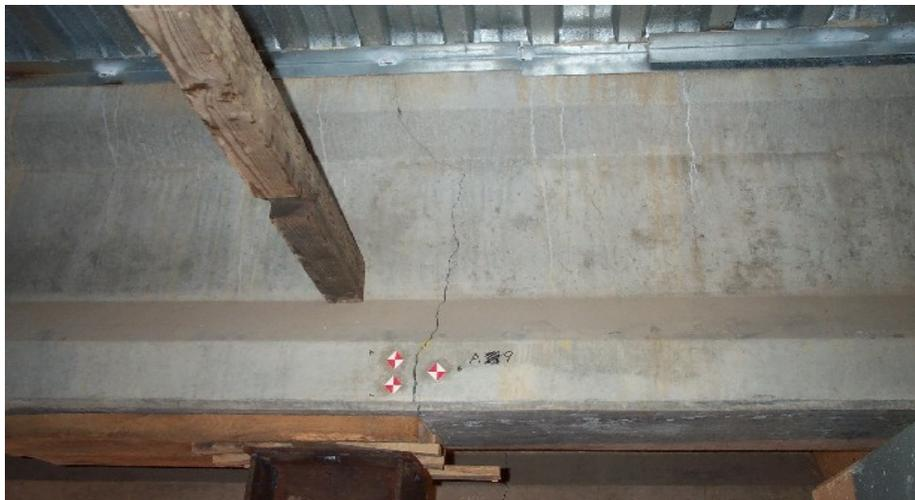
**Figure C30- Cracks near girder supports**
