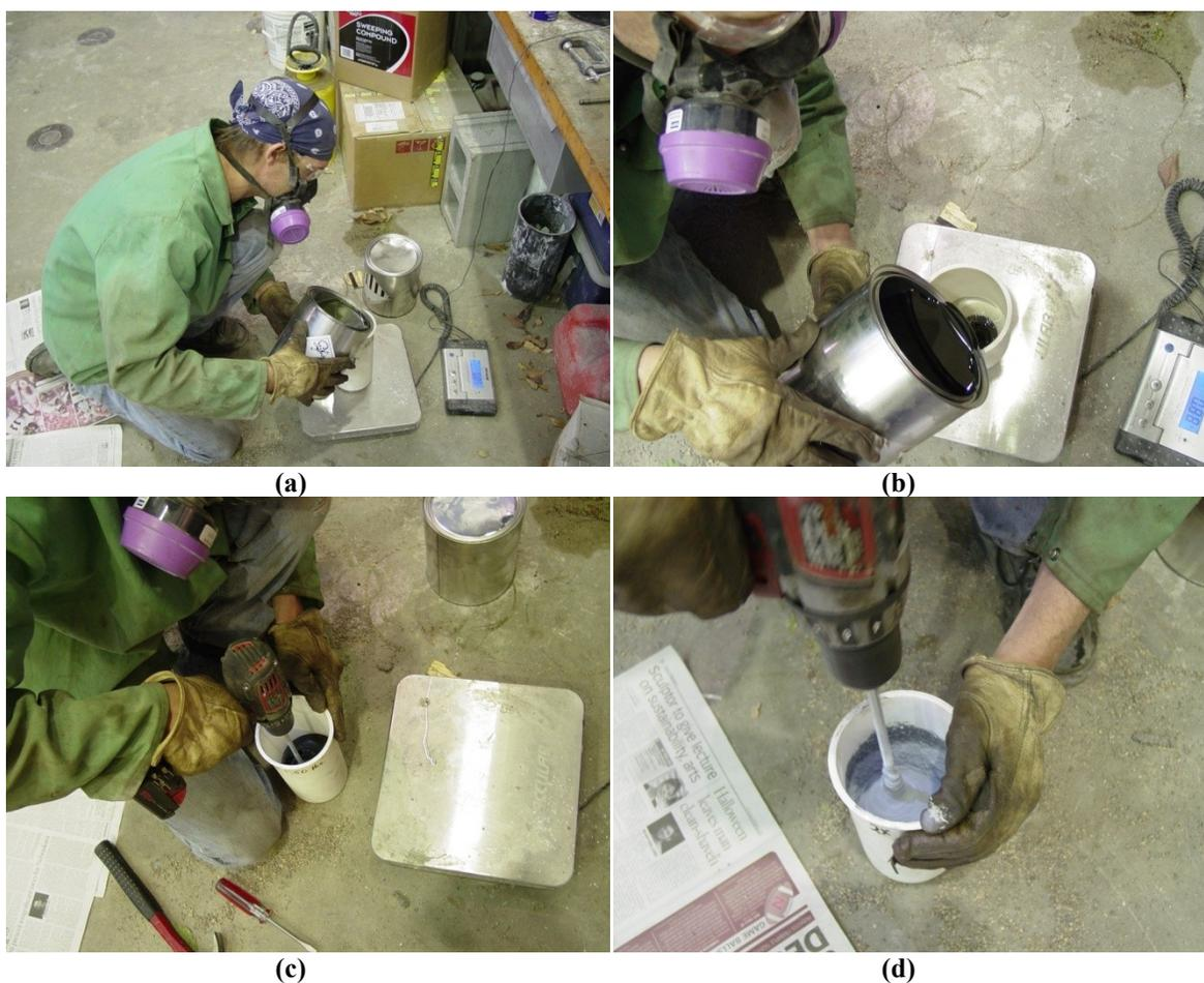
**Figure 4-66- Delpatch mixing procedure**
