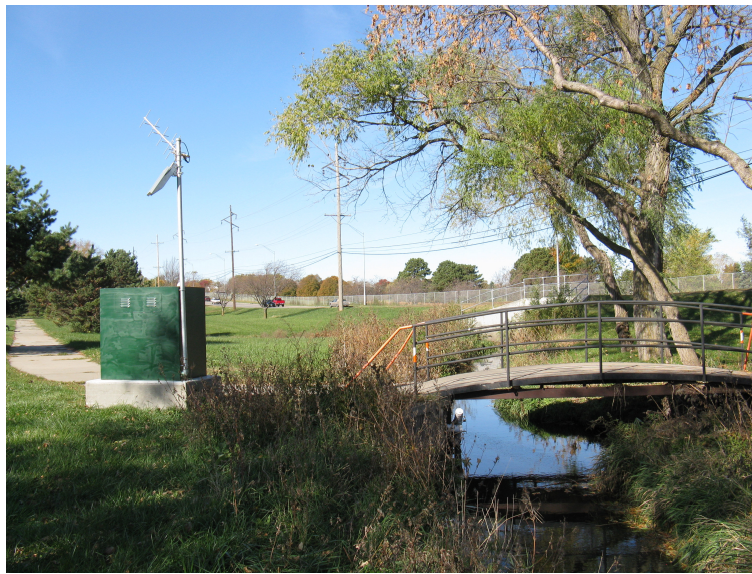
Figure 3.2: Colonial Hills Site in Lincoln, NE, Facing Northwest
