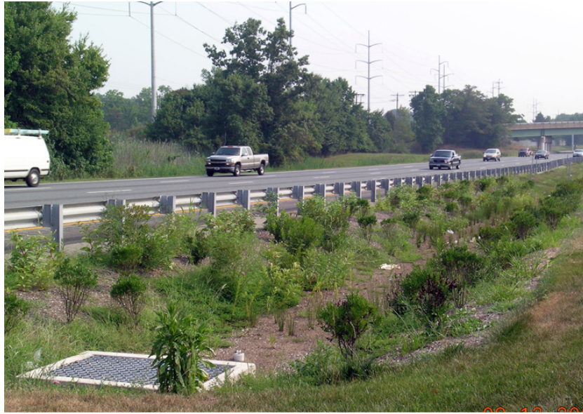
Figure 5 Highway median bioretention in Delaware (DelDOT 2012)
