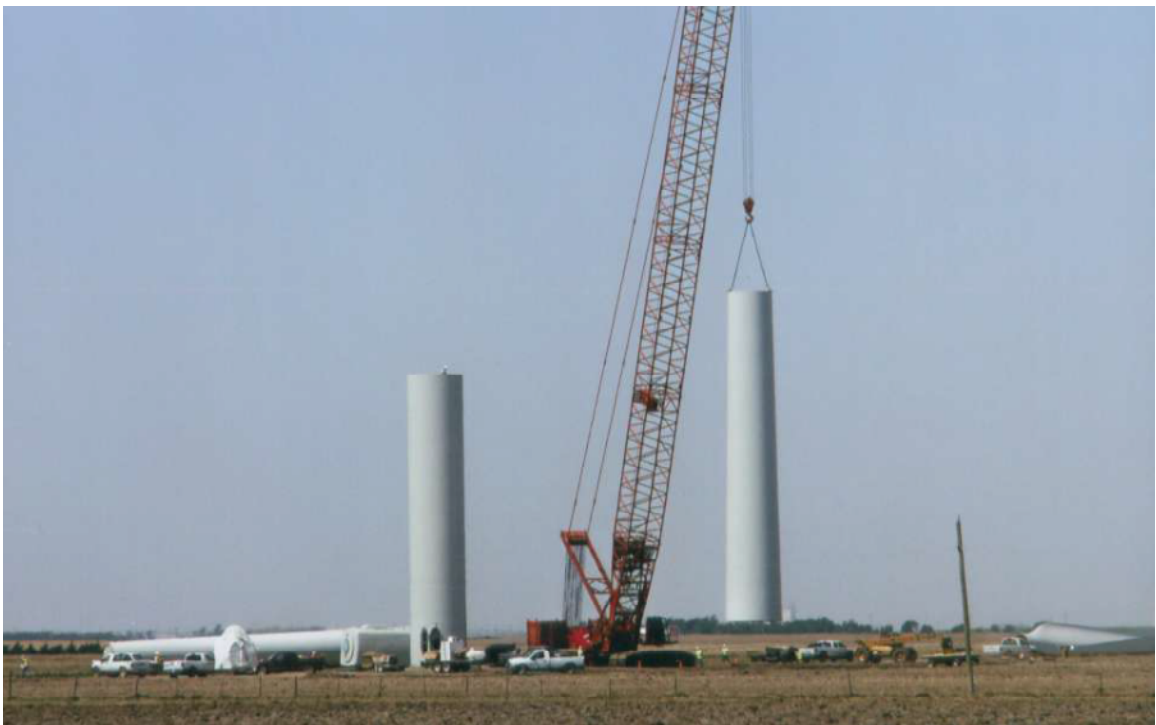
Figure 2-4: Lifting of complete steel tube segments. (Sri, S., 2011)
