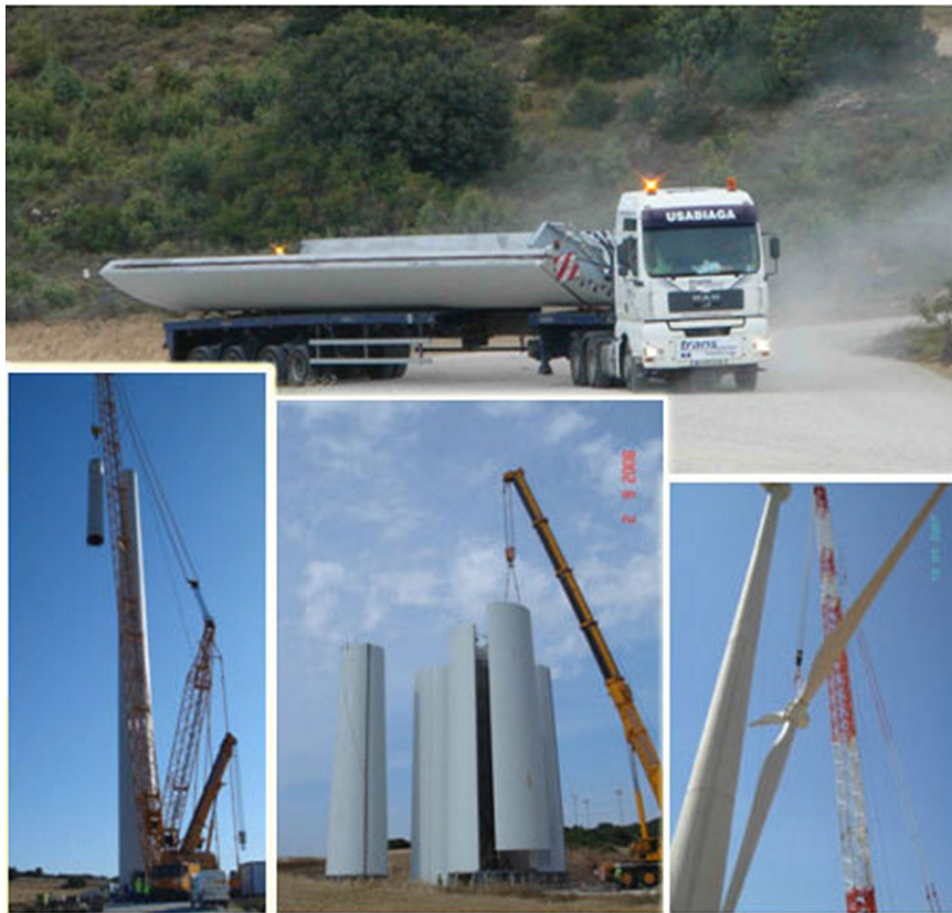
Figure 2-14: Construction of an Inneo Torres tower in Spain. (Jimeno, J., 2012)
