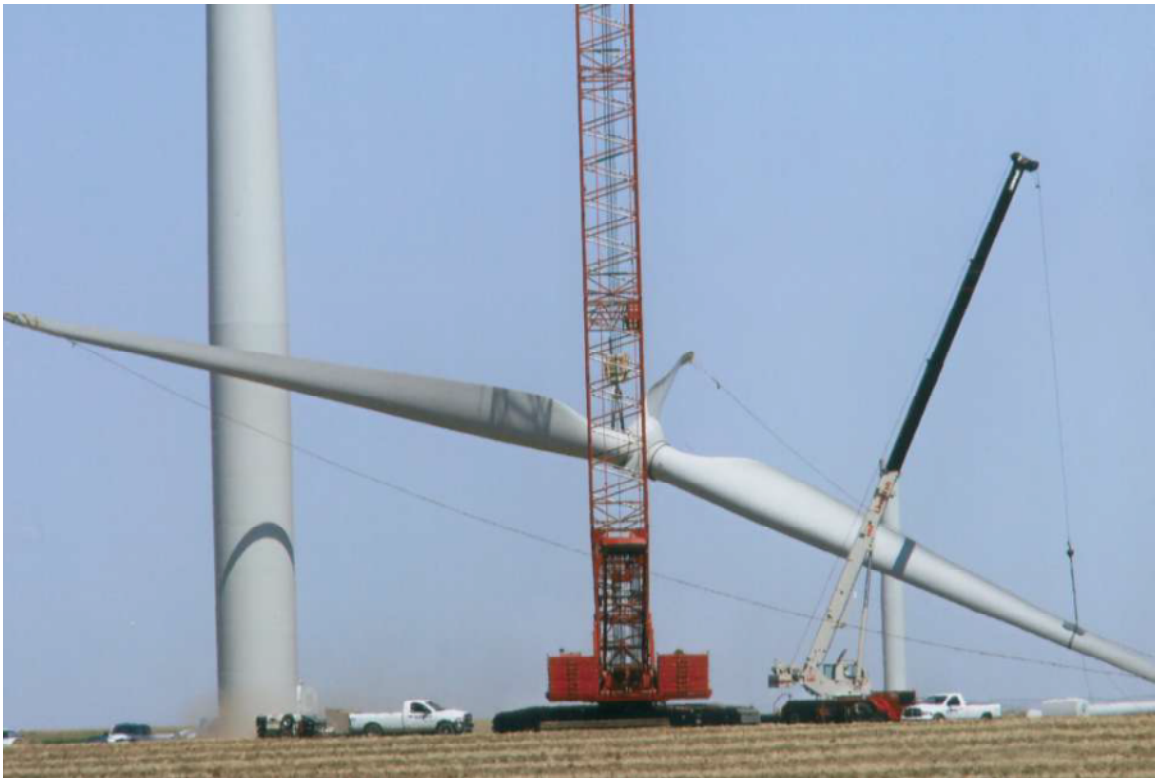
Figure 2-7: Blade tipping using two cranes. (Sri, S., 2011)
