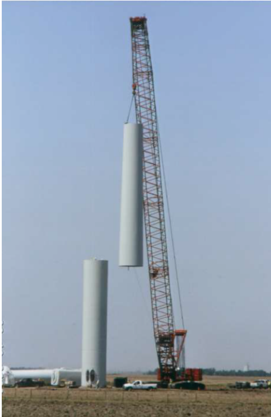
Figure 2-5: Erection of steel towers. (Sri, S., 2011)
