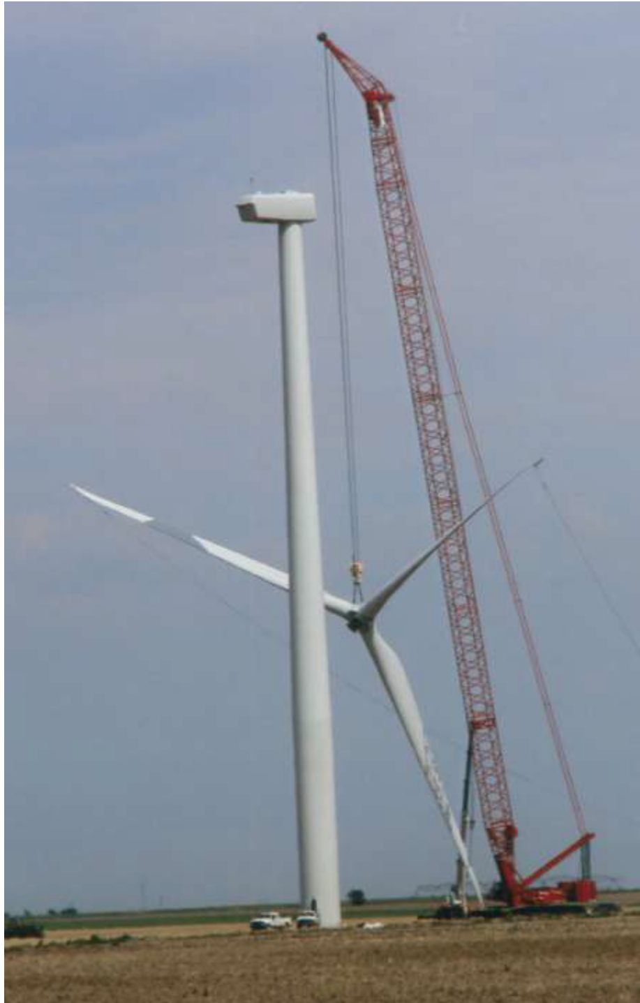
Figure 2-8: Blade lifting using two cranes. (Sri, S., 2011)
