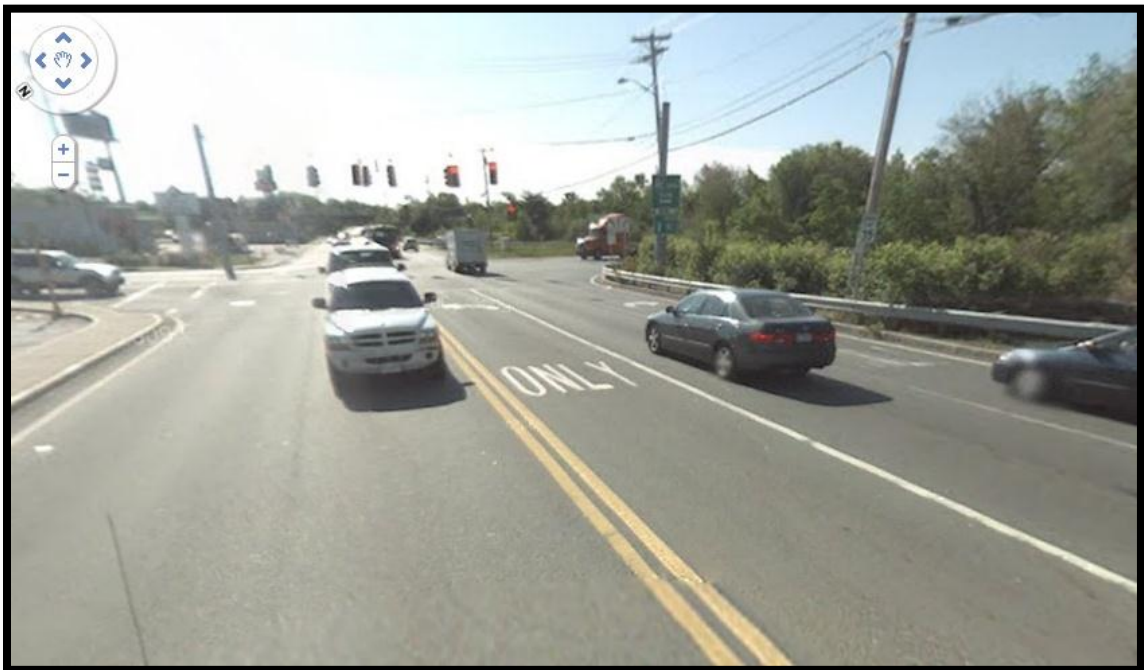
Figure 62. Roadway Segment 242382 – Entrance to I-93 Southbound
