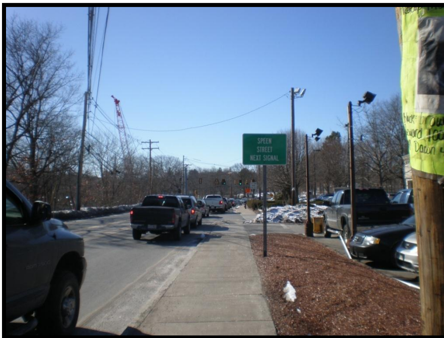
Figure 65. Roadway Segment 259307 – Queue at Intersection of Speen Street
