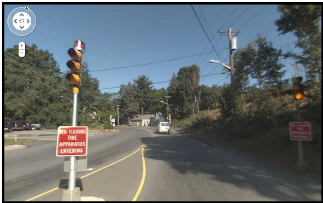
Figure 40. Intersection 201818 - RED FLASHING FIRE APPARATUS ENTERING Signals and Signs
