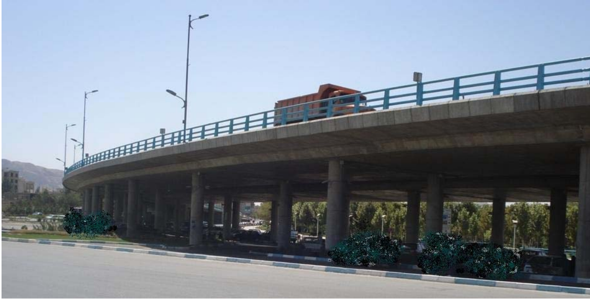
Figure 5.1-1. A Concrete Curved Integral Bridge Similar to the Studied Bridges
