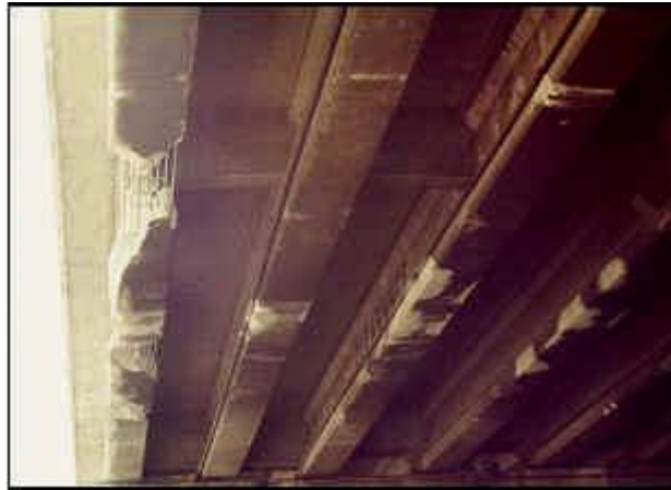
Figure 4.1 Collision Impact on Exterior Girder
