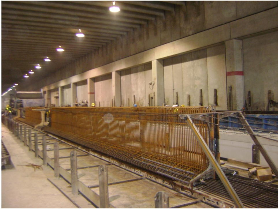
Figure 3.20 NU1100 Reinforcement
