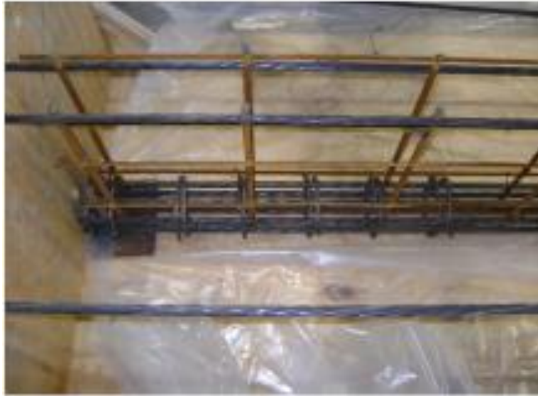
Figure 3.6 T24 End Confinement
