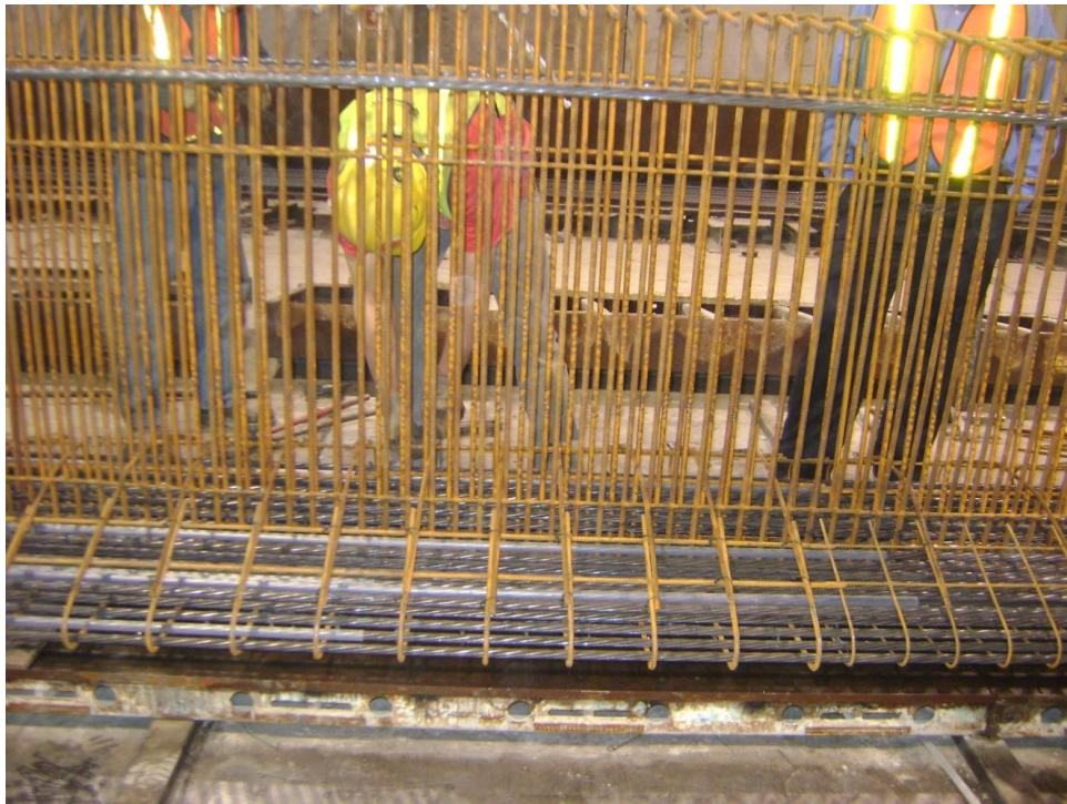
Figure 3.21 NU1100 Confinement Reinforcement
