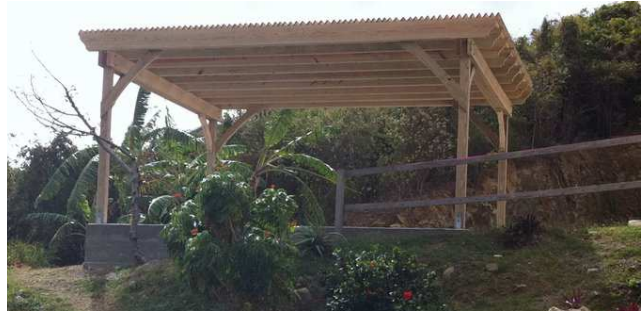
Figure 1. The Outdoor classroom structure is at the top of the terrace gardens. It is used for EARTH classes and for events at the school.
