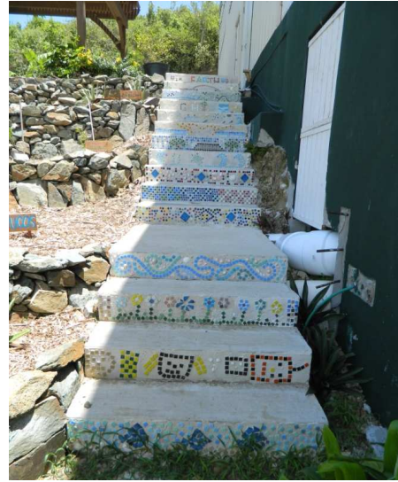
Figure 3. Steps along the side of the terrace garden to the outdoor classroom structure.
