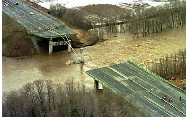
Figure 1.1. Aftermath of Schoharie Creek bridge collapse (Chen, 2011: accessed from http://laser.umkc.edu/~chen/research%20projects.html )
