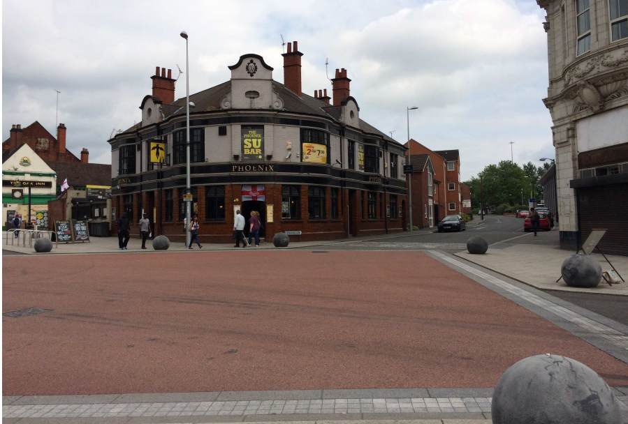
Figure 21: Coventry shared intersection
