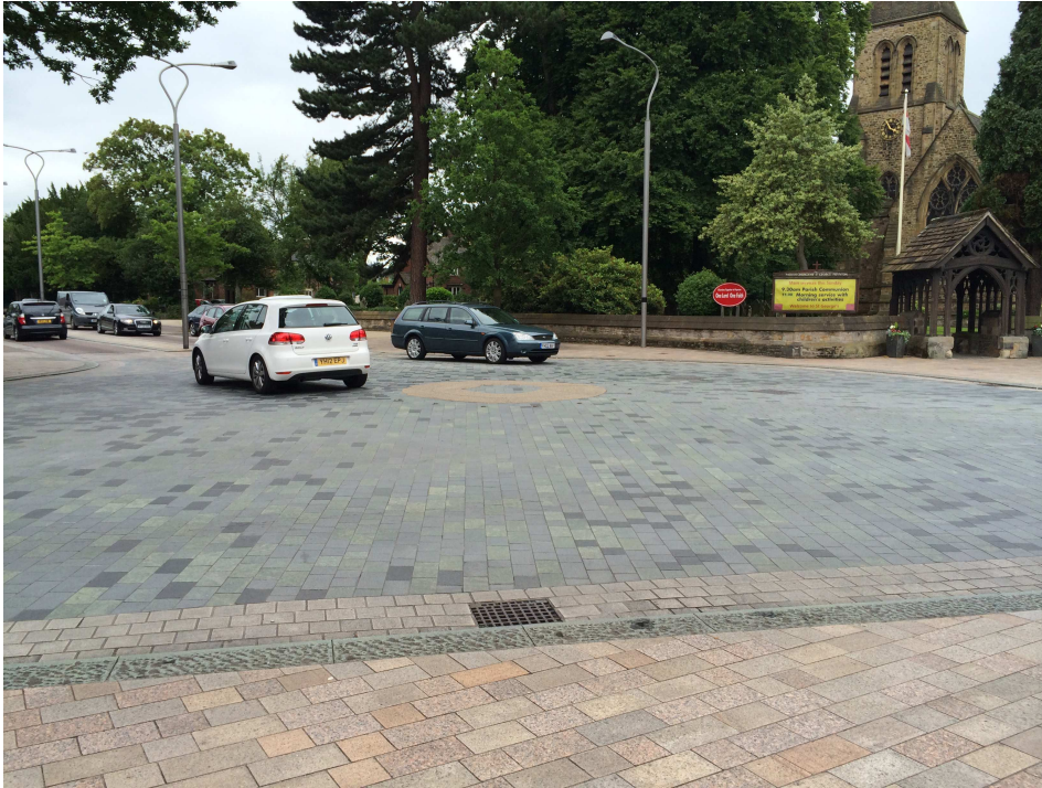
Figure 31: View of Poynton intersection facing southwest
