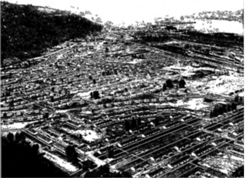
Figure 5-1. (photo) Aerial view of Guild's Lake Courts possibly taken from Montgomery Ward's roof facing Northeast, c. 1944, commissioned by Hal Lidell. Photographer Hugh Ackroyd, who owned and operated a photography studio in Guild's Lake District. Courtesy of Thomas Robinson.
