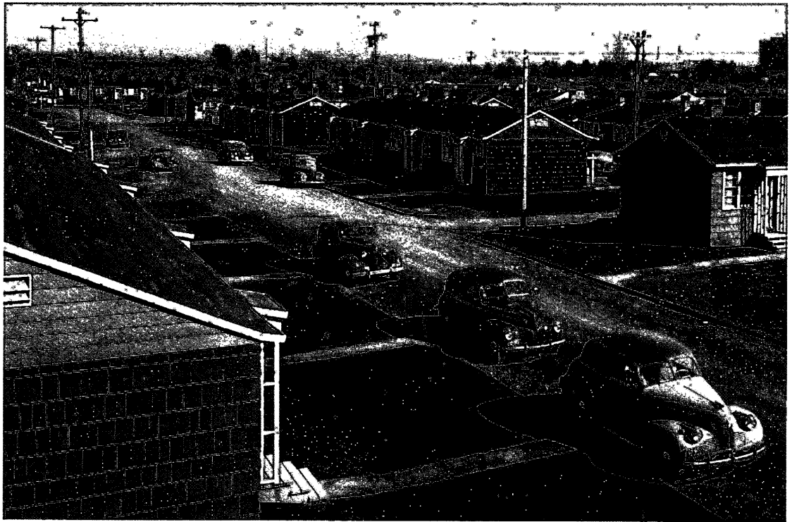
Figure 5-2. (photo cropped) Row houses at Guild's Lake Courts with Montgomery Wards in the distance, c. 1944. Image of units in Guam Court, west of NW 35 th Ave. Photographer Leonard Delano. Courtesy of the City of Portland Archives.
