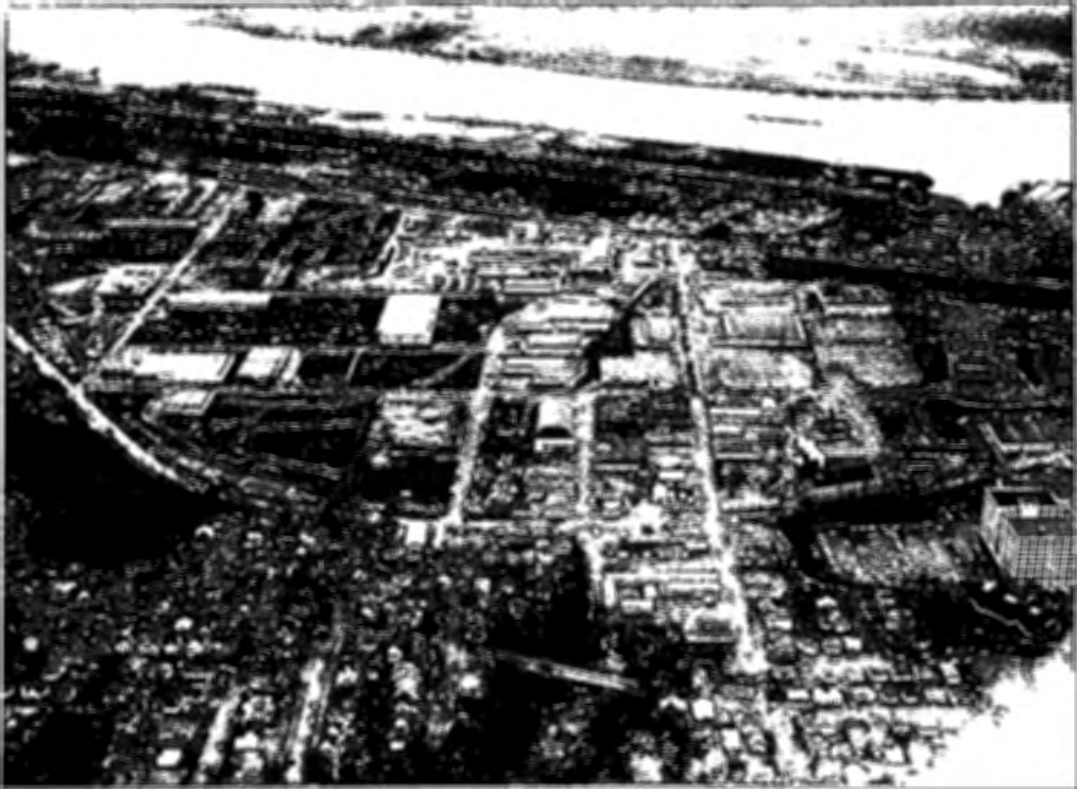
Figure 9-6. (photo) Aerial image taken in 1958 of Guild's Lake District. The area has been transformed into an industrial community with no homes left from Guild's Lake Courts. Courtesy of the City of Portland Archives.
