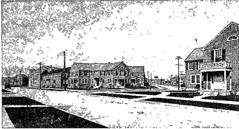
Figure 3-2. (photo) Streetscape c. 1918, Yorkship Village was the first federally funded planned community, designed by Electus D. Litchfield. World War I worker housing near Camden, New Jersey. Courtesy of Frances Loeb Library, Graduate School of Design, Harvard University (#118550).
