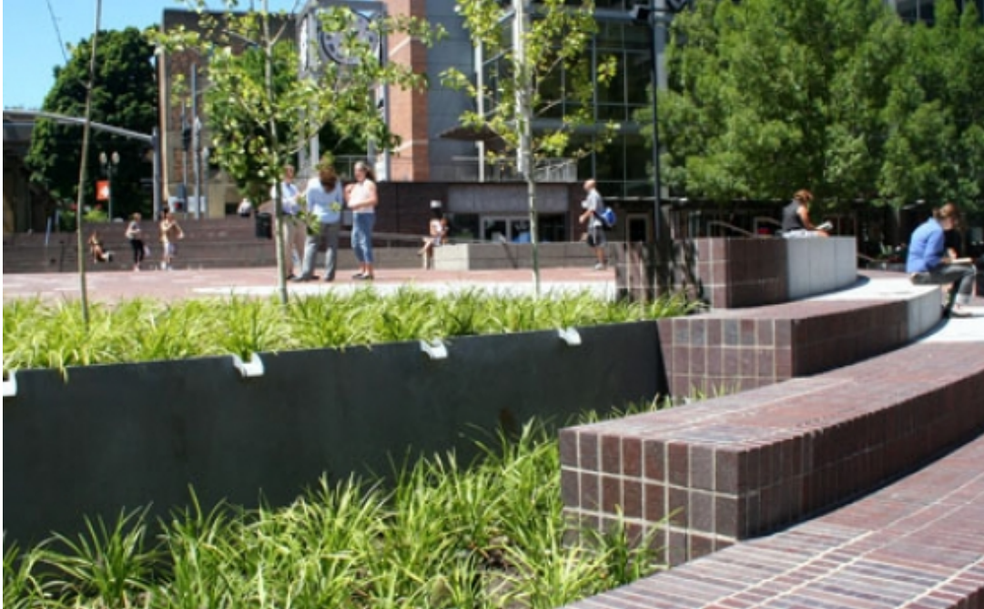
Figure 22: Stormwater retrofit by Nevue Ngan where east steps used to be, part of Phase 3 (“Urban Center Plaza Stormwater Retrofit | Nevue Ngan Associates,” 2011)
