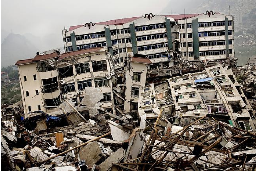
Figure 5. Collapsed Building in 2008 Great Wenchuan Earthquake
