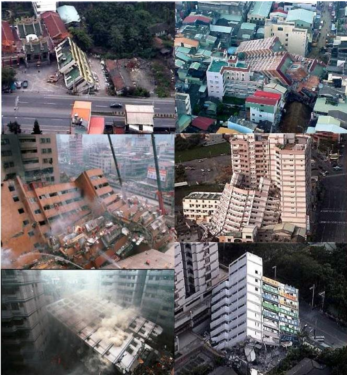
Figure 9. 1995 Kobe Earthquake – Collapsed Buildings
