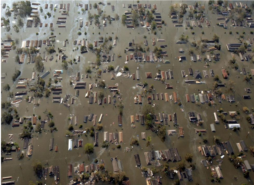
Figure 13. Water Surrounded Downtown New Orleans After Hurricane Katrina 22 .
