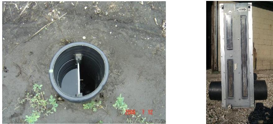
Figure 9 & 10. (Left) The top view of a control gate (managing two different water table heights in the field (Agrem, 2009). Relative control gate size (right)
