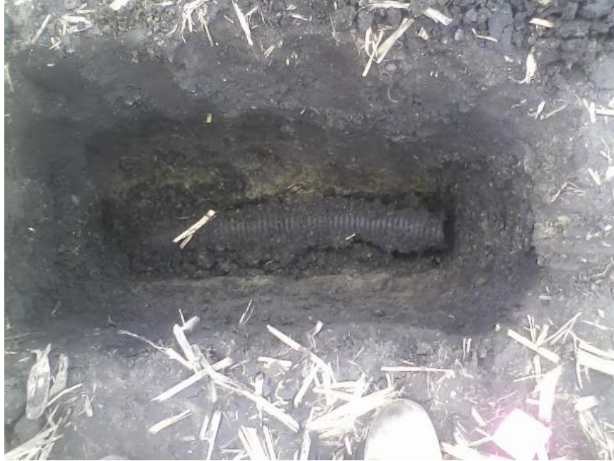
Figure 20. Digging out and cutting of the SI pipes prior to planting
