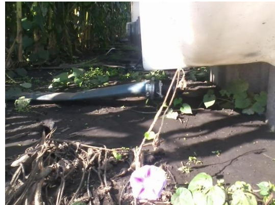
Figure 18. Junction between tank and 1.5 in ID hose
