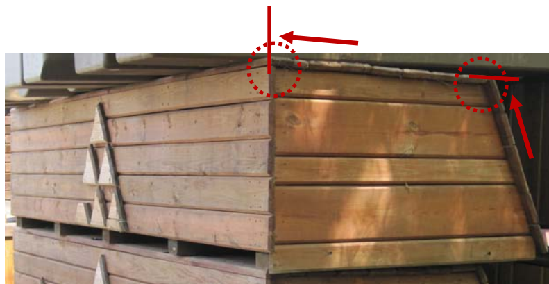
Figure 6.19 Traditional Table Fence Construction
