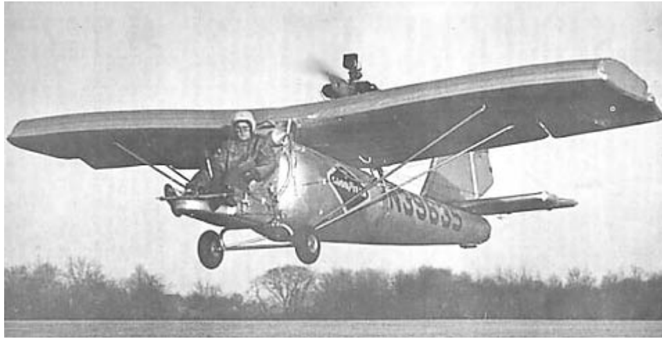
Figure 2.1 – Model GA-468 Goodyear Inflatoplane
