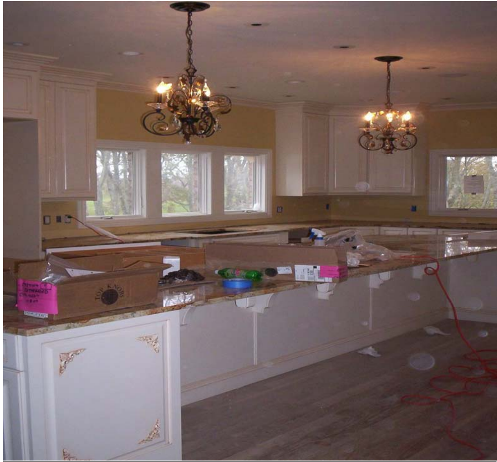
Figure A: Onsite picture 1
