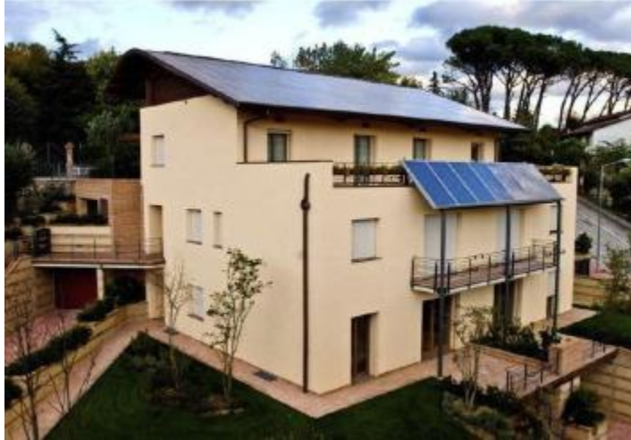
Figure 4. A six-unit apartment microgrid with PV, geothermal, solar thermal, and battery and hot water energy storage (Comodi 2015).
