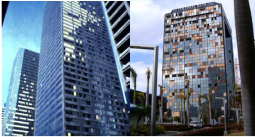
Figure 1. Building Damages during Hurricane Alicia in 1982 (left) and Hurricane Wilma in 2003 (right), by Beers [1]
