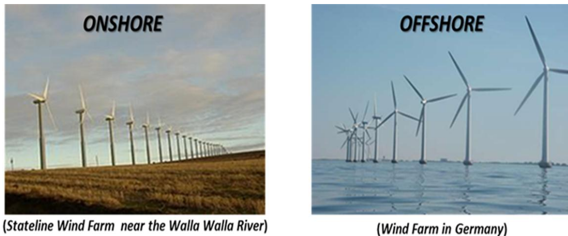
Figure 1-11 Onshore and offshore wind farms
