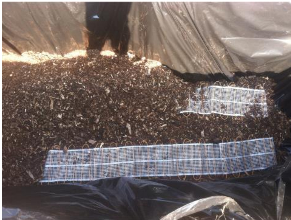
Figure 9. Installation of ThermoTile underground heaters
