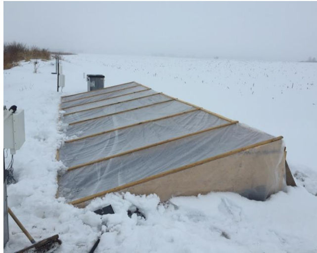
Figure 12. Passive solar heater in operation
