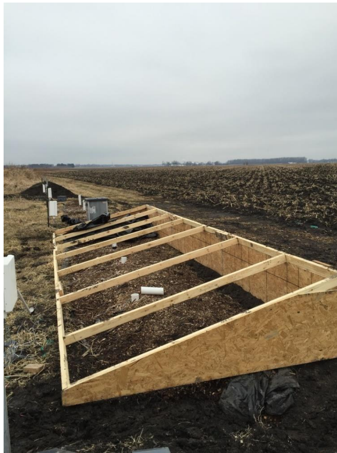
Figure 11. Passive solar heater during construction
