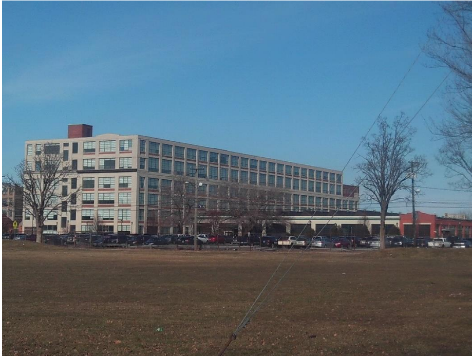
Figure 21. South Armory building
