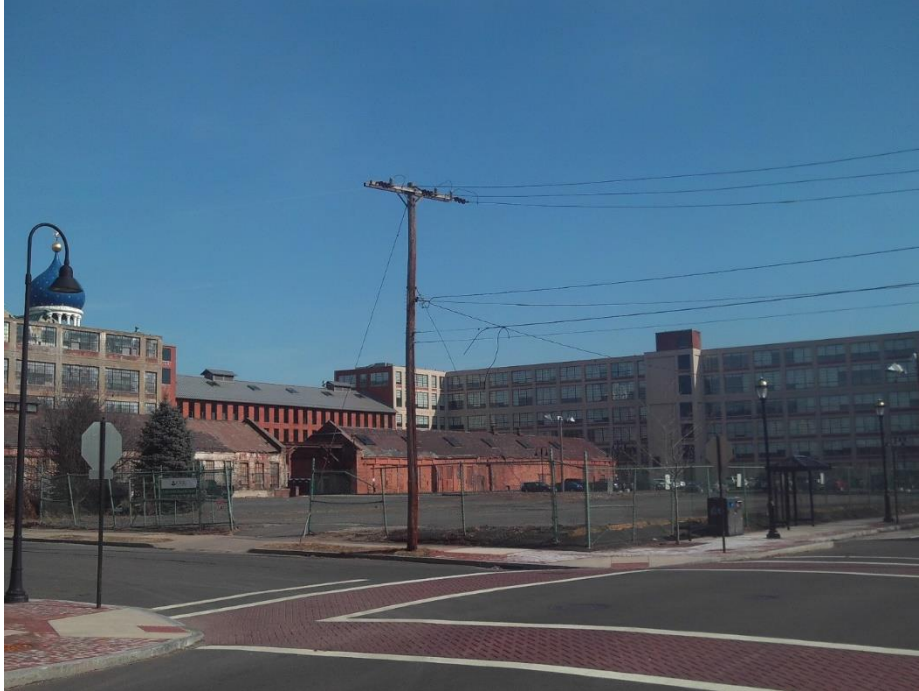
Figure 7. View of the factory complex from Huyshope Avenue and Sequassen Street. The still-unrestored Foundry and Forge Shop, the low buildings in the foreground, are slated to house the future visitor center and museum (Gosselin 2016).
