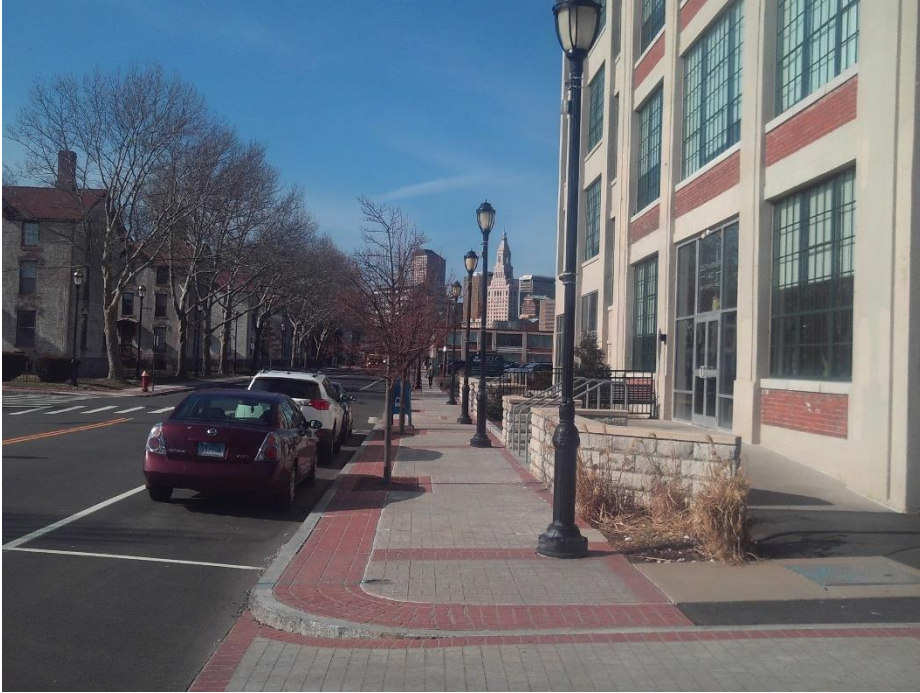
Figure 23. South Armory building (right) and worker housing (left), Huyshope Avenue, view toward downtown Hartford
