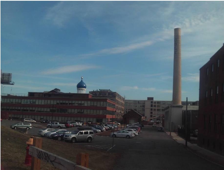
Figure 10. View of the factory complex from the north; photo taken from Van Dyke Avenue near Vredendale Avenue, looking southward.
