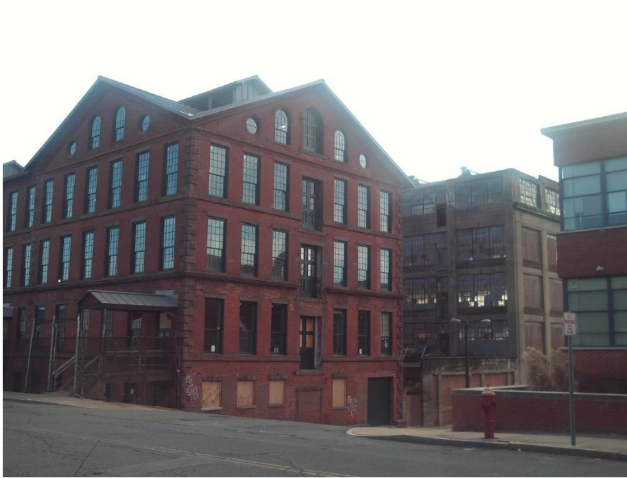
Figure 15. Corner of East Armory (foreground, left), North Armory (background), and U-Shaped (office) building, Van Dyke Avenue at Sequassen Street
