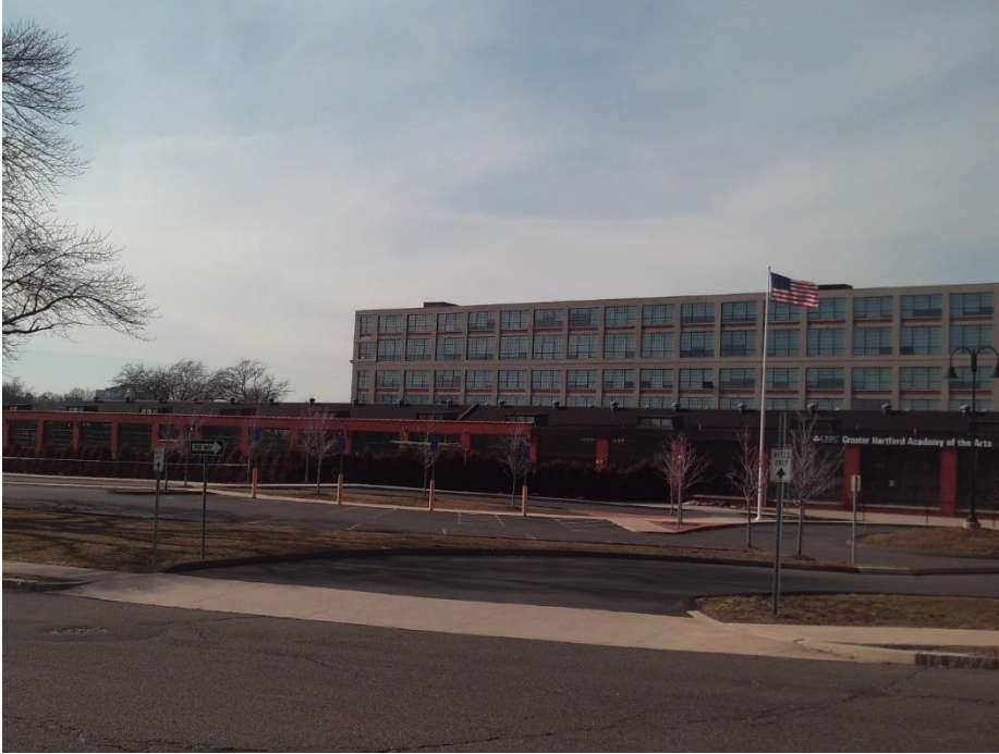
Figure 9. The south side of the former factory, the Machine Shop (foreground) and East Armory (background). Taken from Masseek Street between Van Dyke and Huyshope Avenues.
