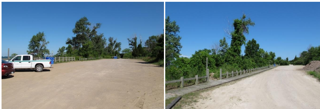
Figure 1.1: 2009 photos showing boardwalk in NW beach of Point Pelee. The site had formerly been dunes prior to the parking lot construction. The photos show the extent of damage (photo courtesy: Dr. M-L Byrne).
