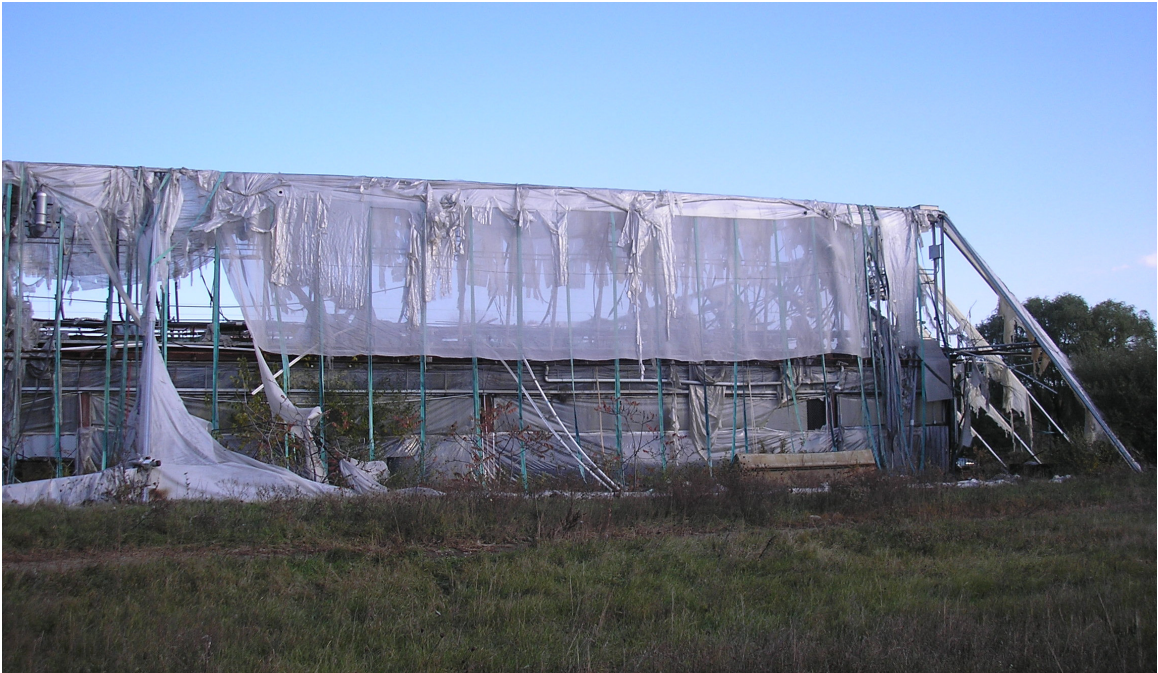
Figure 8: Current state of the Bioshelter
