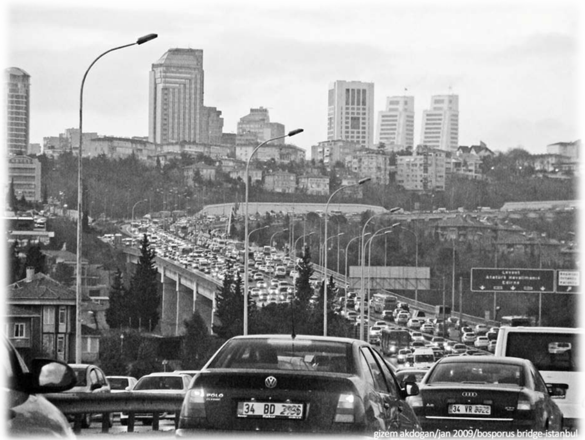
Figure 1- Congested traffic in the European landing of the Bosphorus Bridge. Photo by Gizem Akdoğan.
