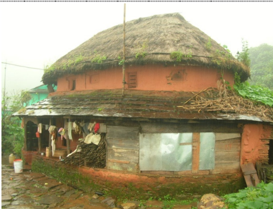
Figure 4.3- A typical Gurung house Source: By Gaurav Tuladhar
