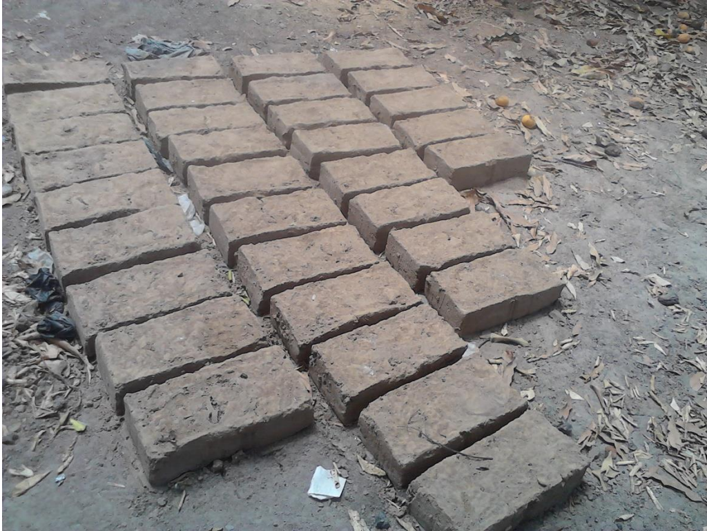
Figure 2.13: Gambian Earth Blocks: Newly cast earth blocks curing in open air in a construction site in The Gambia
