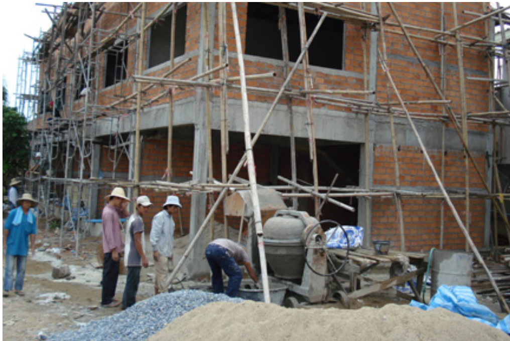
Figure 4: Thai modern architecture: construction with column and beam concrete and brick masonry wall
