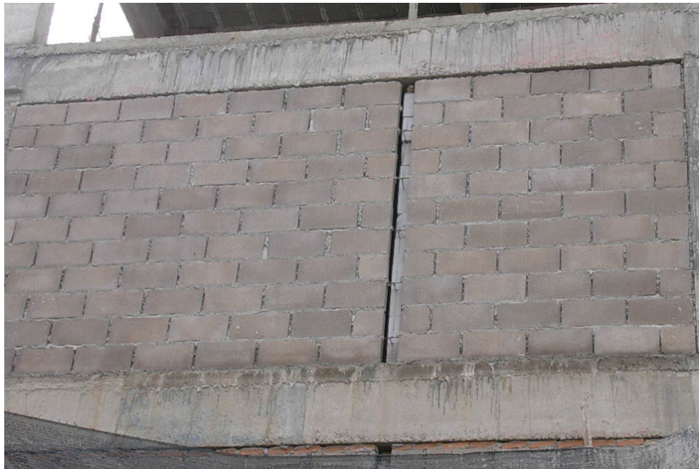
Figure 20: Concrete masonry unit or concrete block wall
