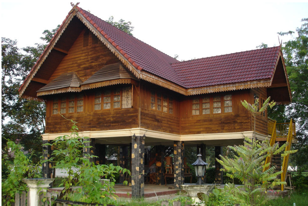
Figure 8: Contemporary Thai Northern style house where wood is still preferred. The structure is half concrete and half wood.
