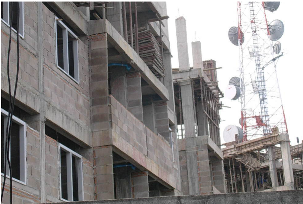
Figure 22: Concrete block construction
