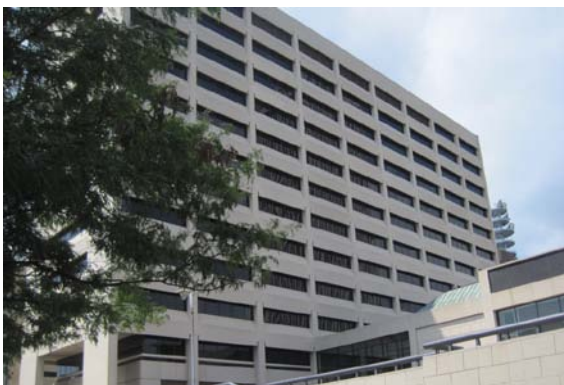
Outside view from south east
