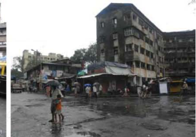
Low to Medium cost housing provided by MHADA, Maharashtra Housing Area Development Authority
