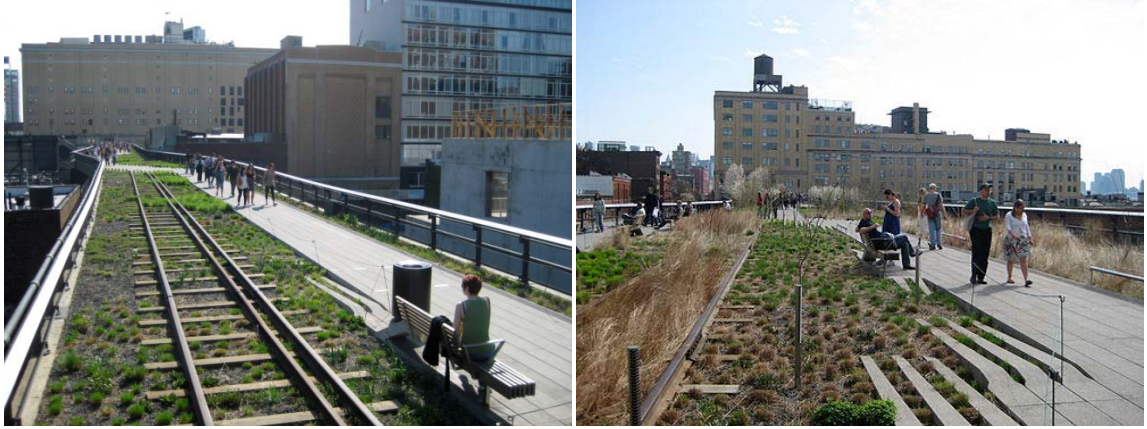
Figure 56 2 : Highline rail bridge, Figure 57 3 : Highline Park features
