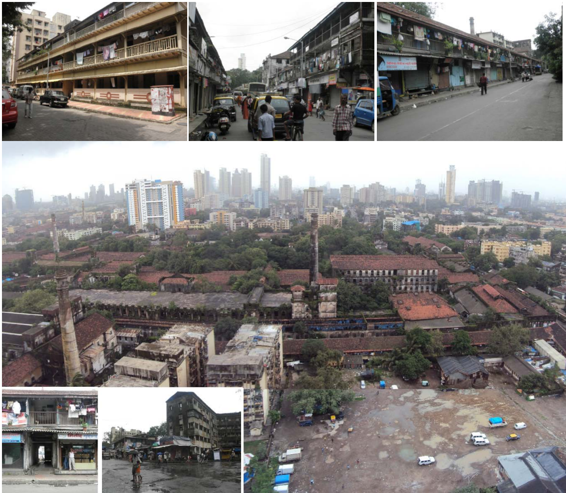
Figure 45: Mill workers housing (Author)
