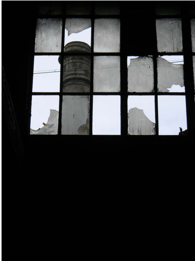
Figure 63: Mill Chimney (Author)
