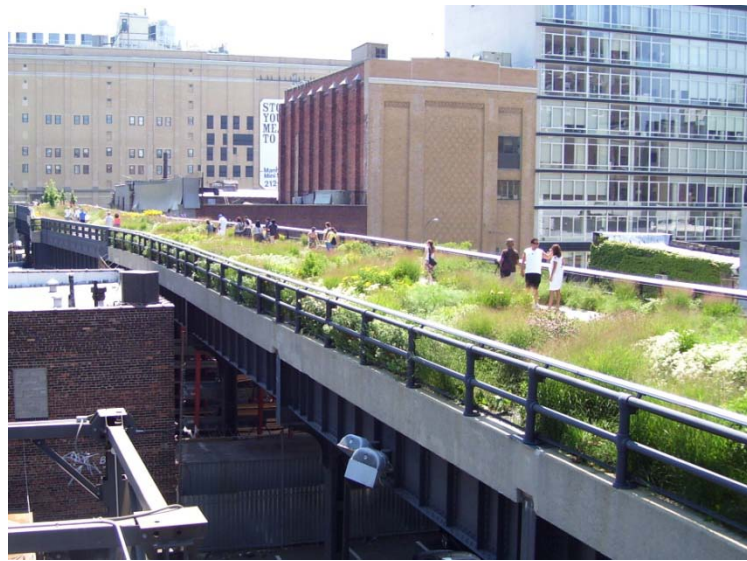
Figure 55: Elevated Highline Park 1
