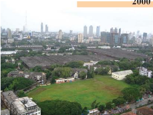
Figure 19 14 : Aerial view Parel, Mumbai Mill land redevelopment, Reclamation salt pan lands and Mangrove forests.
