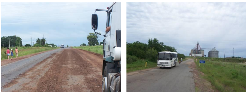
Figure 6- Secondary roads in the outskirts of Mercedes. Photography by author
