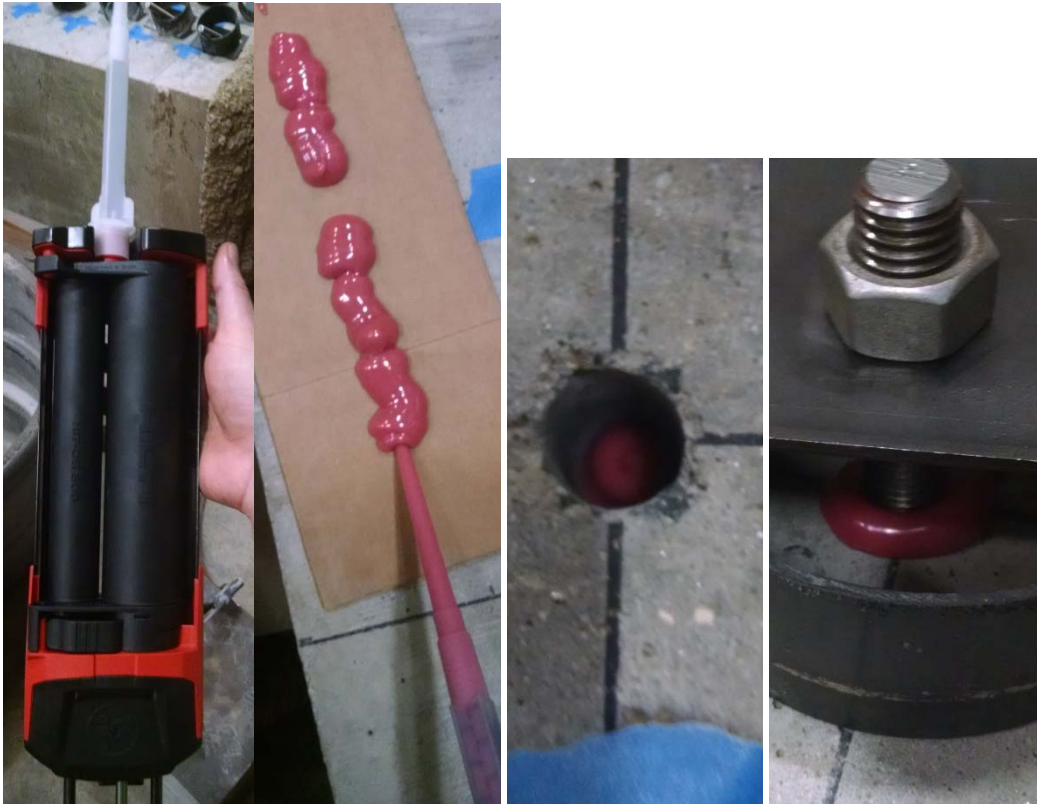
Figure 8.9 Adhesive Application
