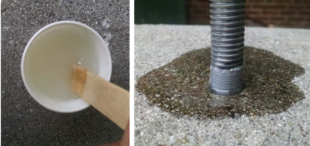
Figure 8.4 Mixed Epoxy (Left) and Installed Anchor (Right)
