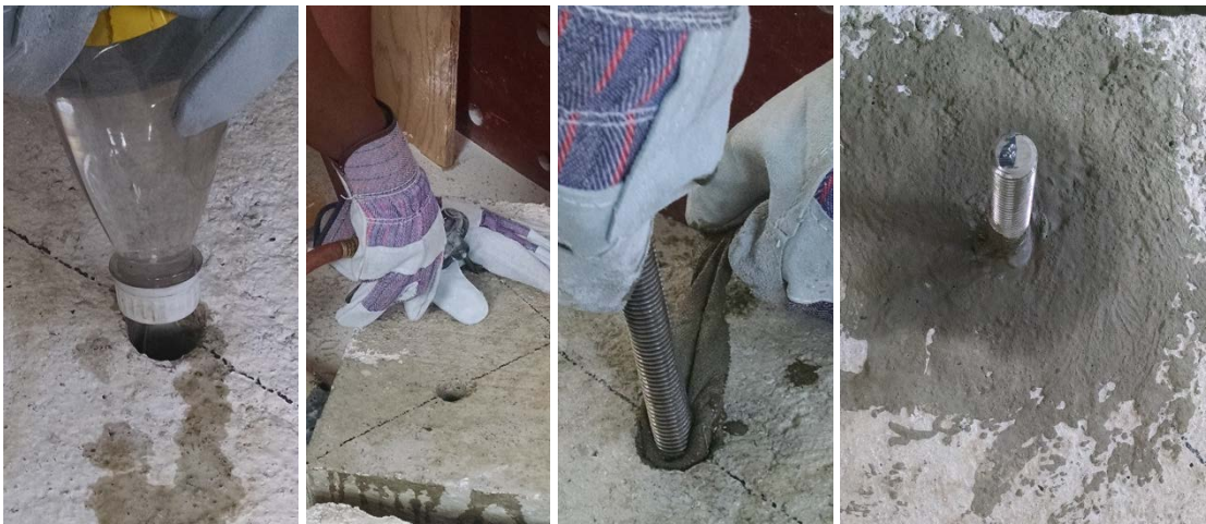
Figure 8.11 Test Series 0c Installation Photos.
