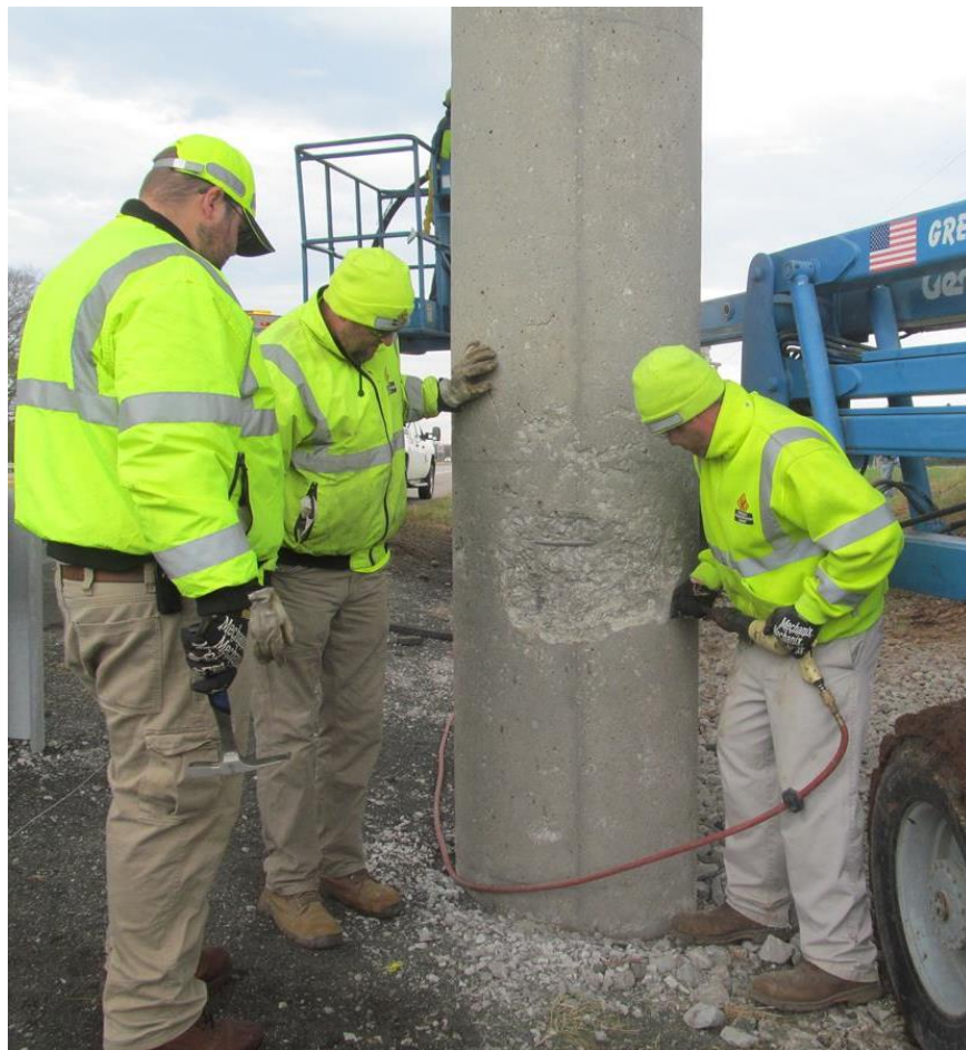
Figure 5.15 – Removing loose concrete material
