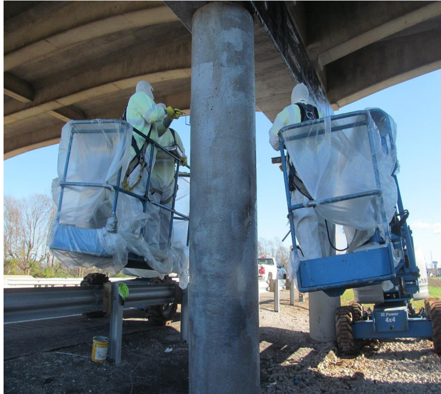
Figure 5.17 – Application of primer coating on the concrete surface
