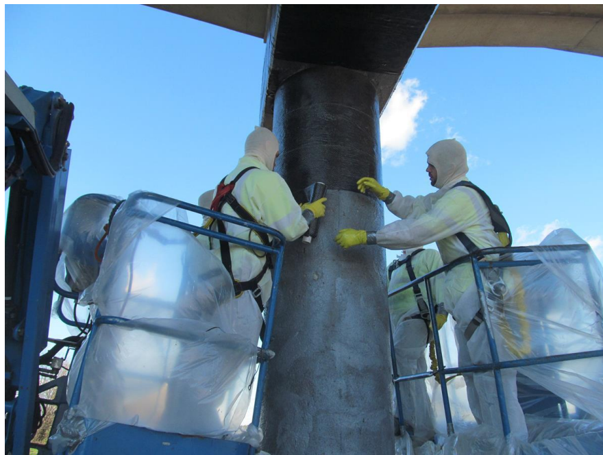
Figure 5.18 – Application of Unidirectional Carbon Fabric
