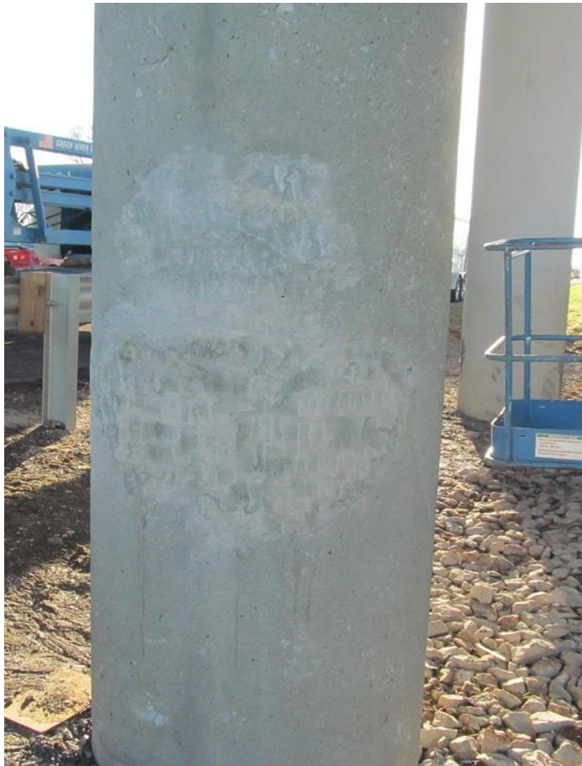
Figure 5.16 – Placement of repair mortar
