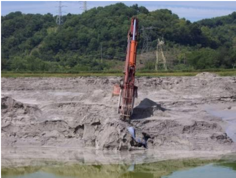
Figure 1.15: Trackhoe engulfed in fly ash at the DPL impoundment after a fly ash failure caused by liquefaction
