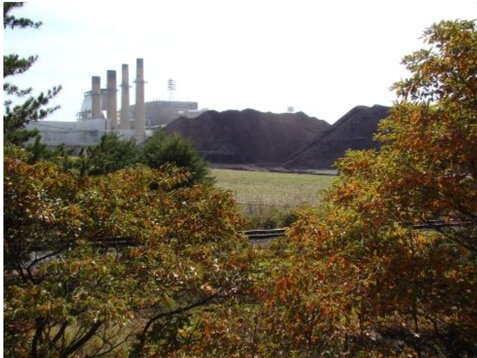
Figure 1.5: Dry disposal storage in a coal ash landfill
