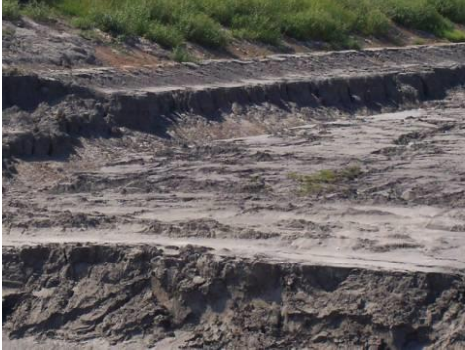
Figure 1.14: Movement of fly ash at the DPL impoundment
