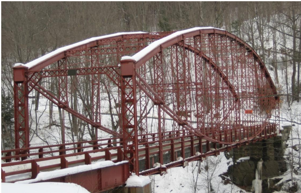
Figure 8.1 – Photograph of Bardwell's Ferry Bridge.
